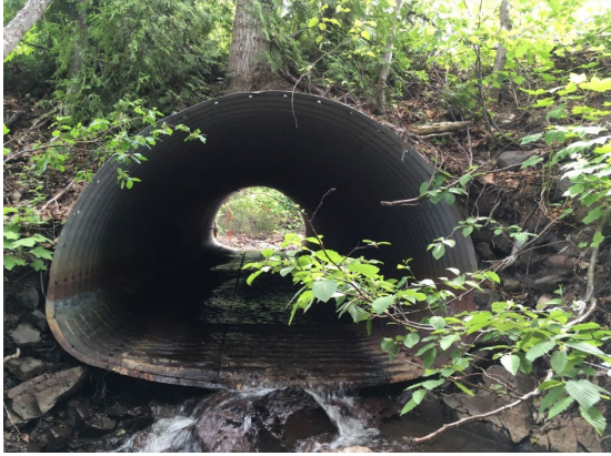
The Razor parking lot culvert, with cedar swamp habitat, looking downstream.
