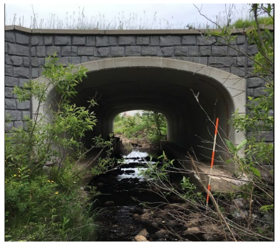
The Walmart culvert, a concrete arch with wingwalls, looking upstream.
