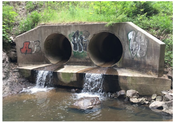
The Calverley Ave. culvert a, two barrel concrete culvert, looking downstream.
