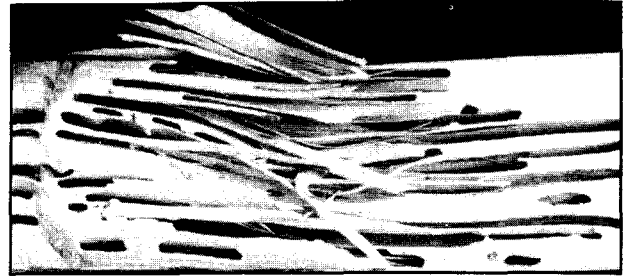
Figure 6. Damage caused by carpenter ants
