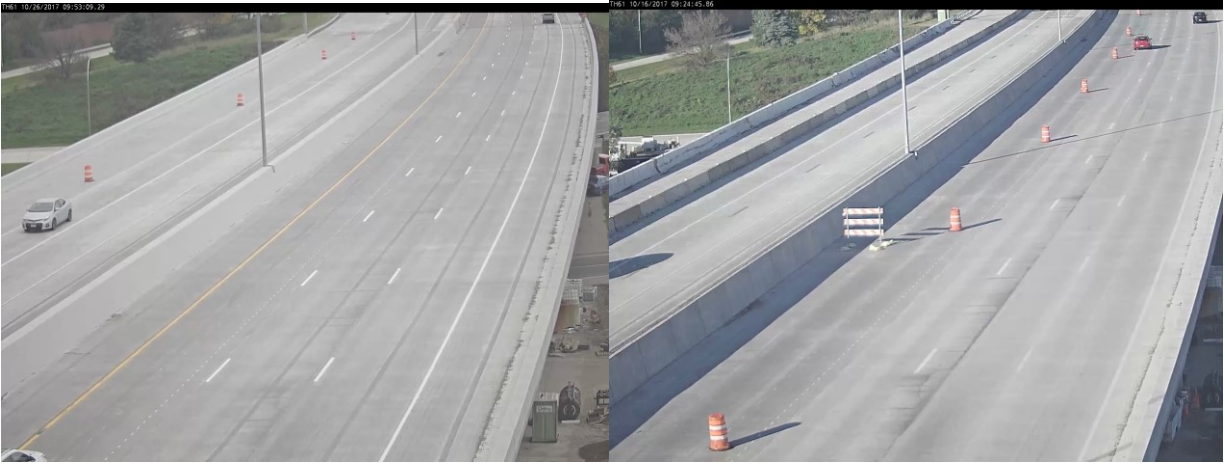
Figure 5.10 TH-61 Station. All Lanes Open. Normal Road, 3-lane No Shoulder
