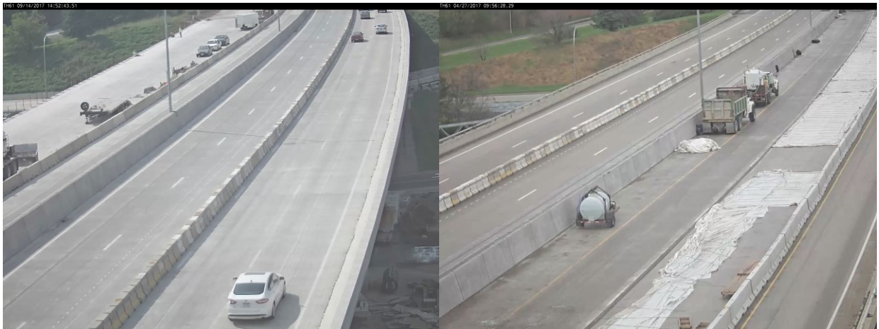
Figure 5.11 TH-61 Station. Reduced Lanes Layouts. 2-Lane No Shoulder, 2-Lane No Shoulder Through only
