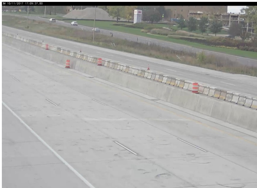
Figure 2.25 Camera view for the camera at 3M station in 2017
