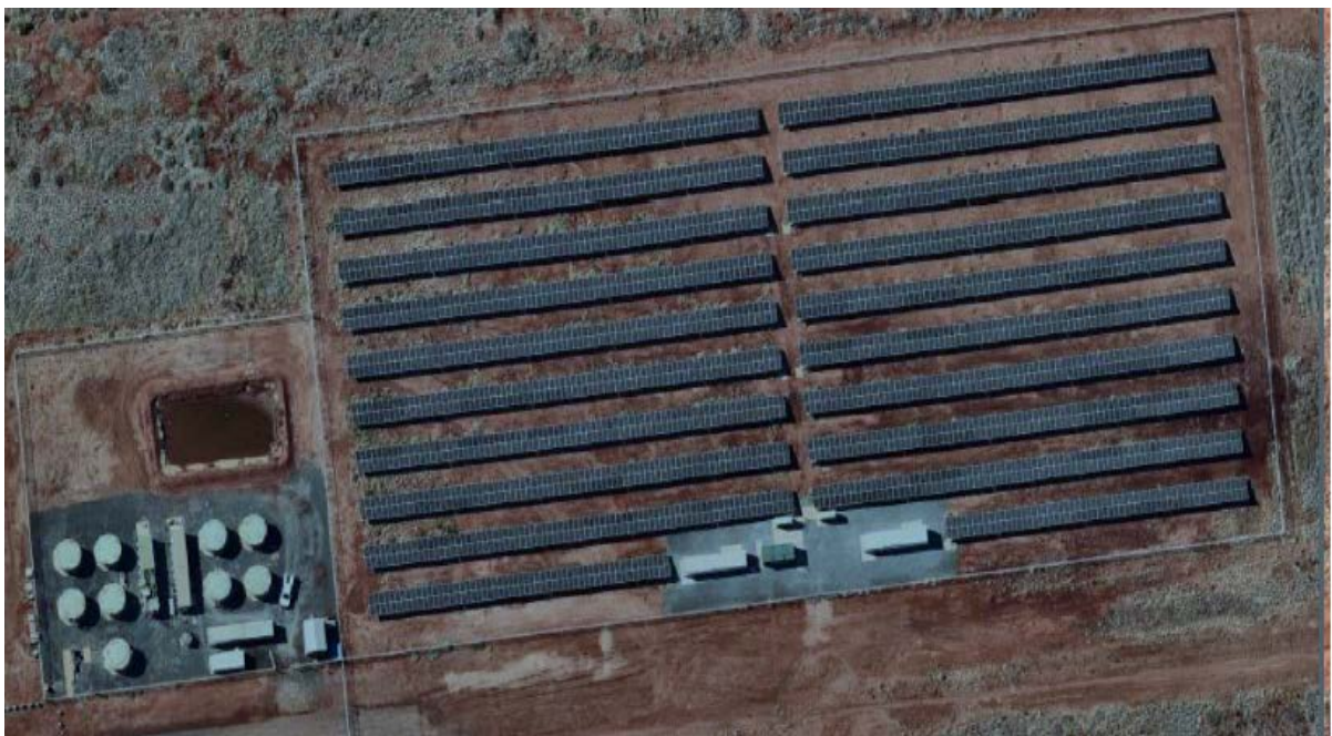
Fig 3.5 Aerial view of Karratha Airport PV plant (Harris 2018a).
