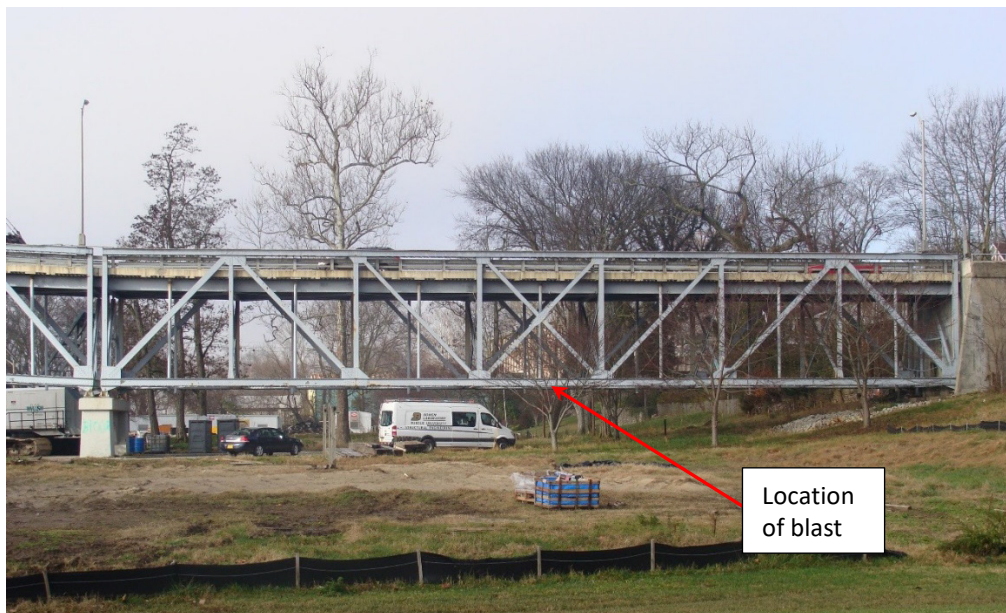
Figure 2.3 Approach span of Milton Madison Bridge tested for redundancy
