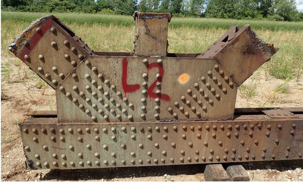
Figure 4.47 Example of deeply set two-channel diagonal members connected into a gusset plate
