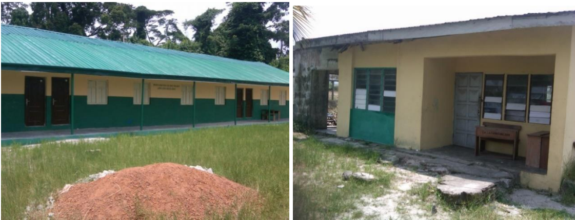
Figure 5.9: Refurbished Classroom block and the staff building
