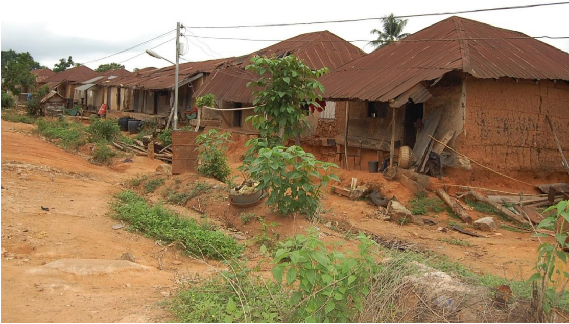
Figure 5.18: Low Voltage lines at Onibambu Village
