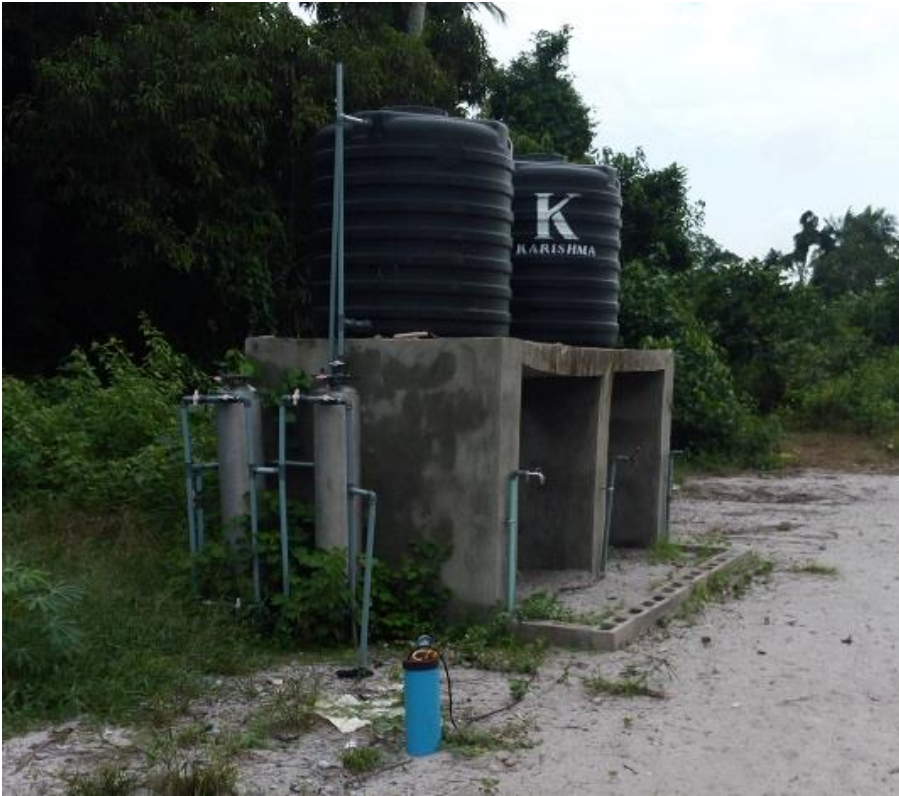
Figure 5.14: Gasoline generator powered water borehole under construction
