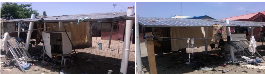
Figure 5.16: The dilapidated and non-functional Solar-Powered System at Sagbokoji Settlement
