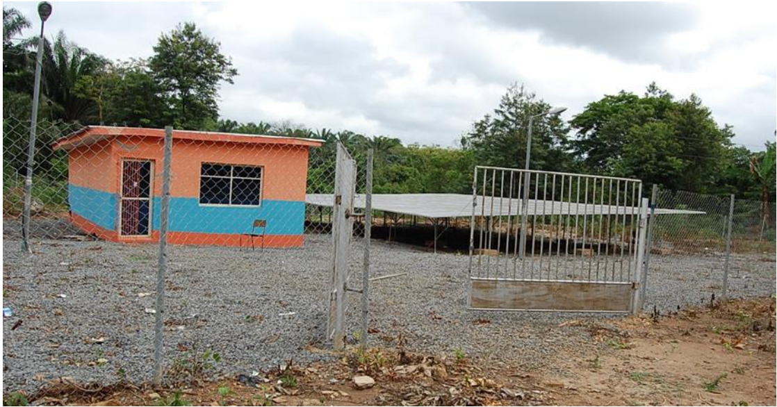
Figure 5.17: The Solar Array
