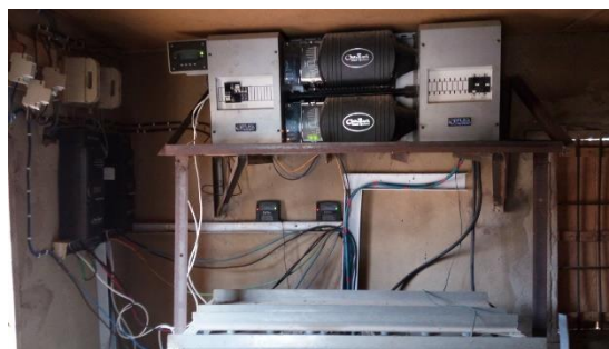
Figure 5.22: The Control House and Balance of System Equipment in the Control Room
