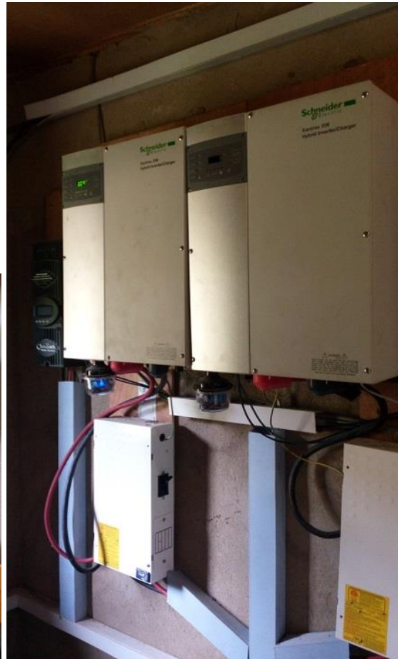
Figure 5.27: Balance of System Equipment in control room at Umuode Community
