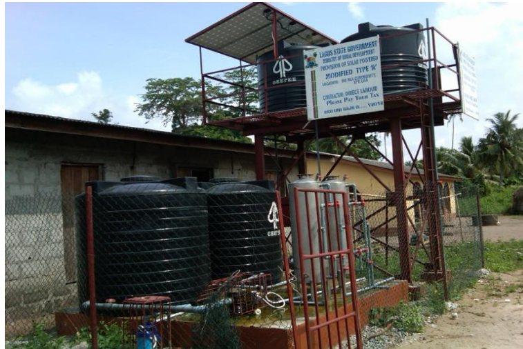
Figure 5.7: Installation at Ide I
