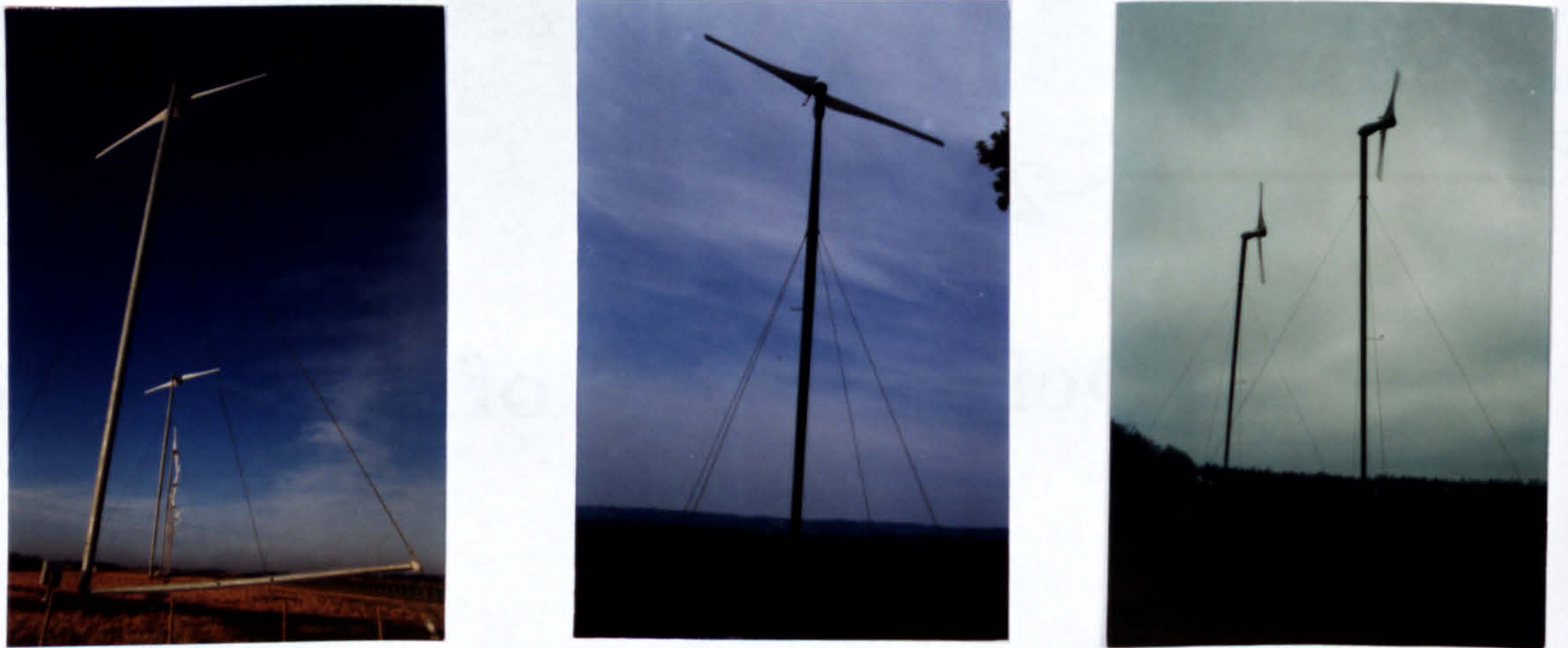
Figure 2.1: The three wind turbines studied: the Carter 300 kW machine at Great Orton Airfield (50 m tower), the Carter 300 kW machine at Facombe Estate (39 m tower) and the Carter 25 kW machine at West Beacon Farm (15 m tower).
