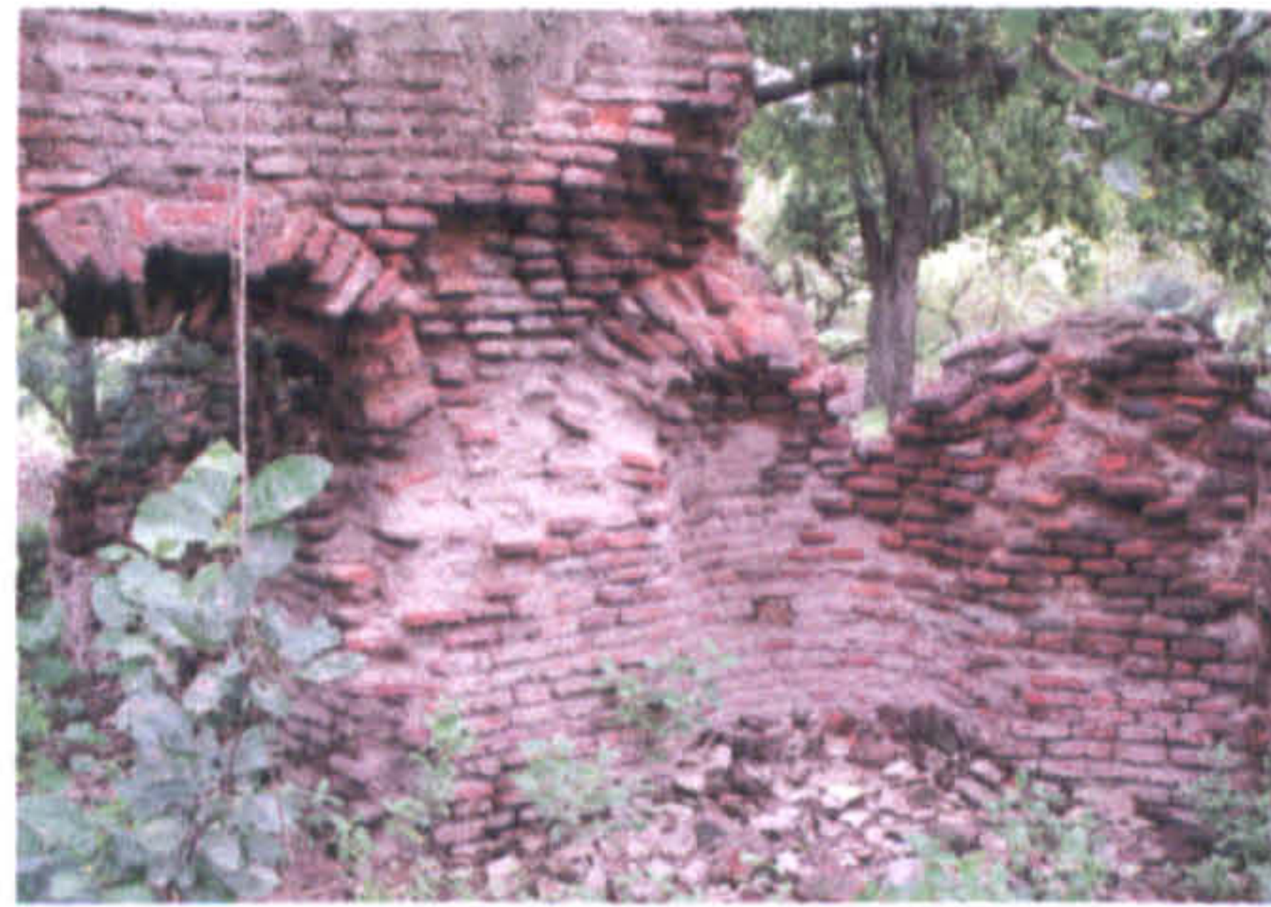
Fig.2.19a Probable remnants of Metcalfe Sahib-ki Kothi-I
