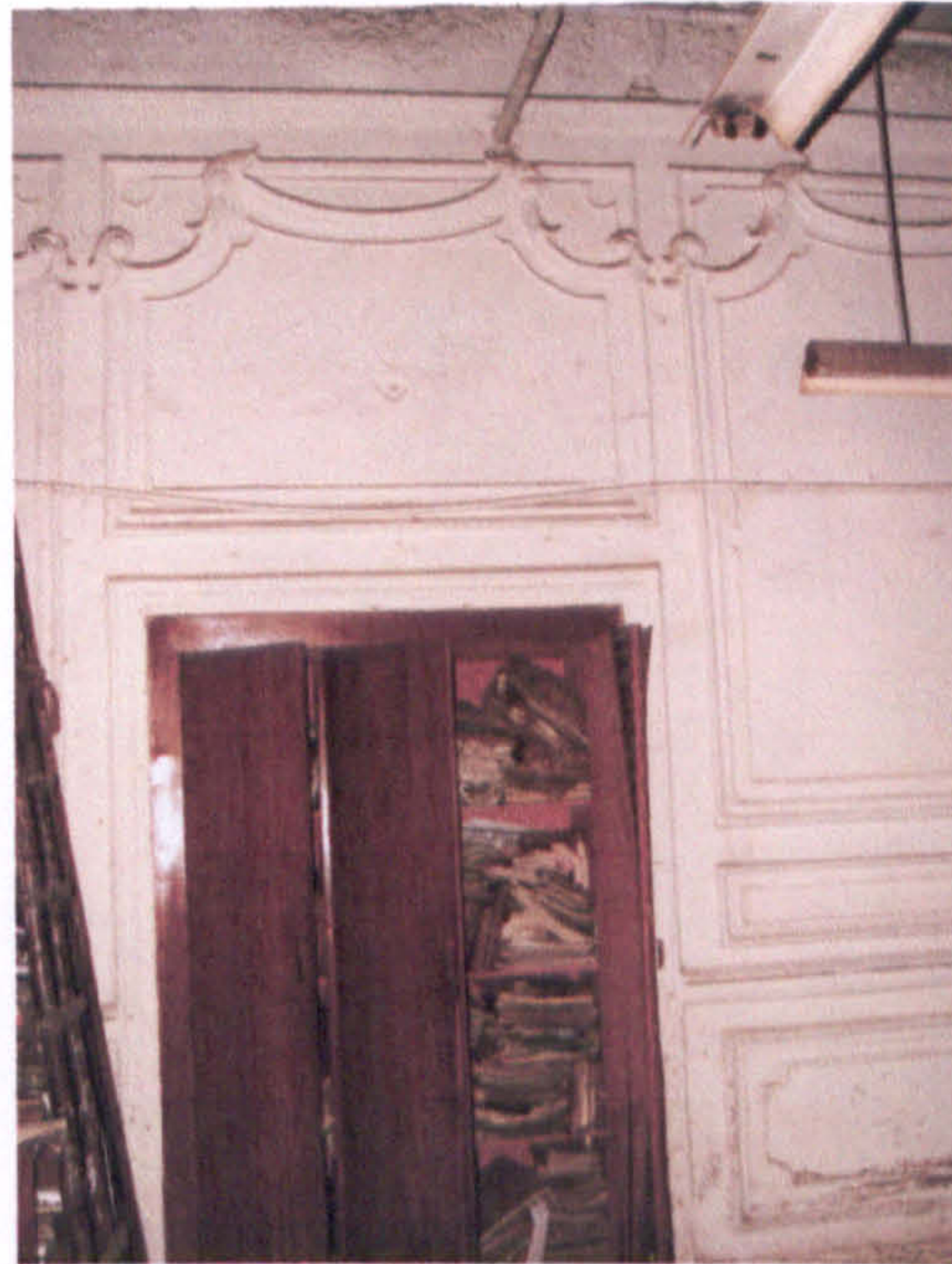
Fig.8.8h The Kothi: a side chamber with stucco ornament-II
