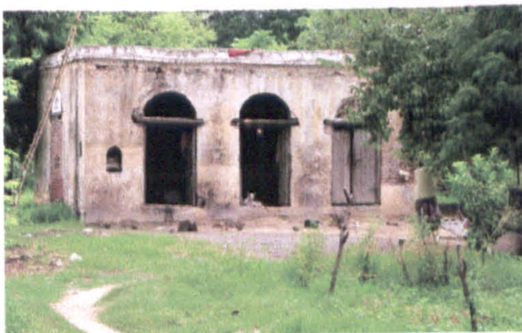
Fig.2.8a Surviving service building
