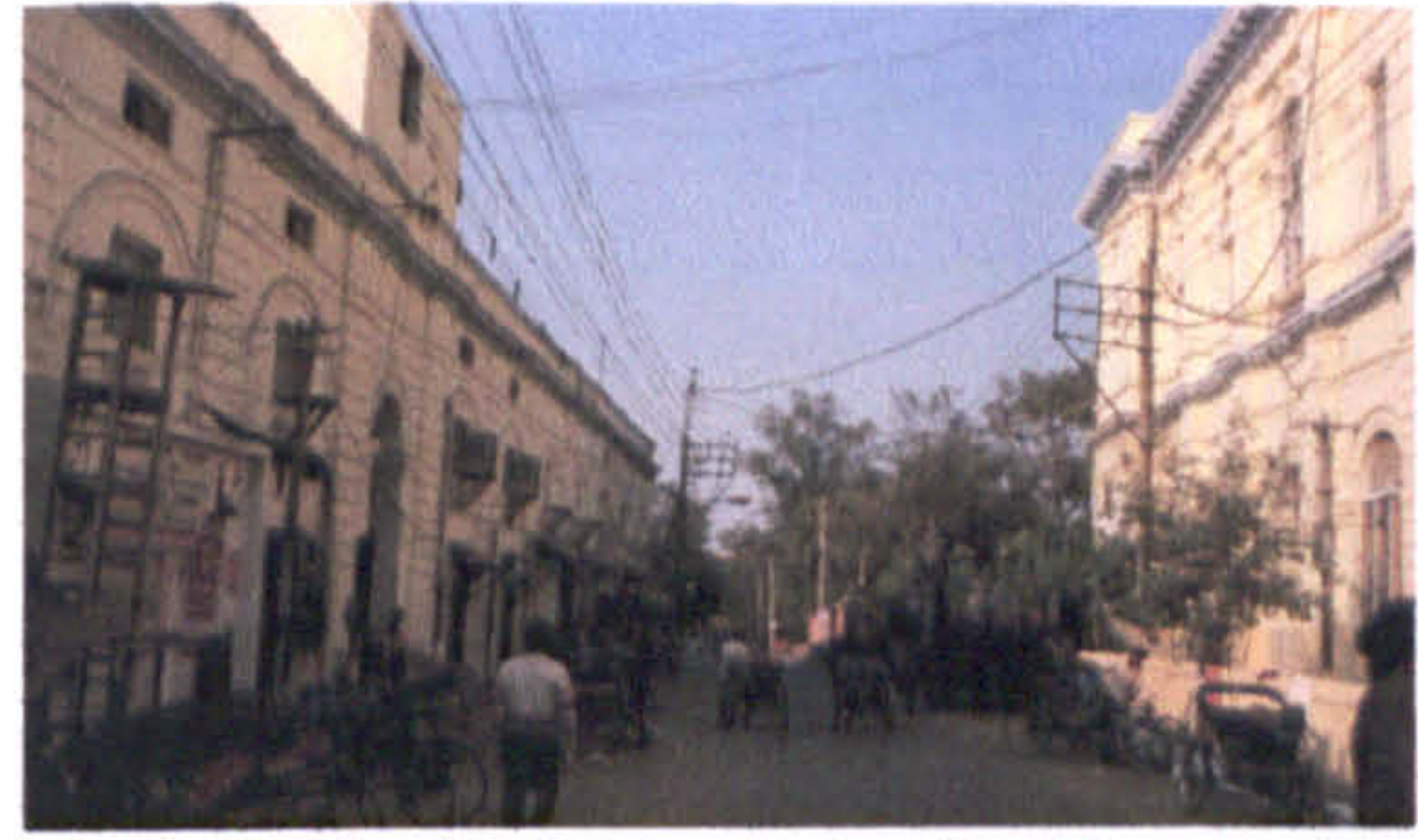
Fig. 1.3b The Delhi Institute: flanking ancillary structures-II
