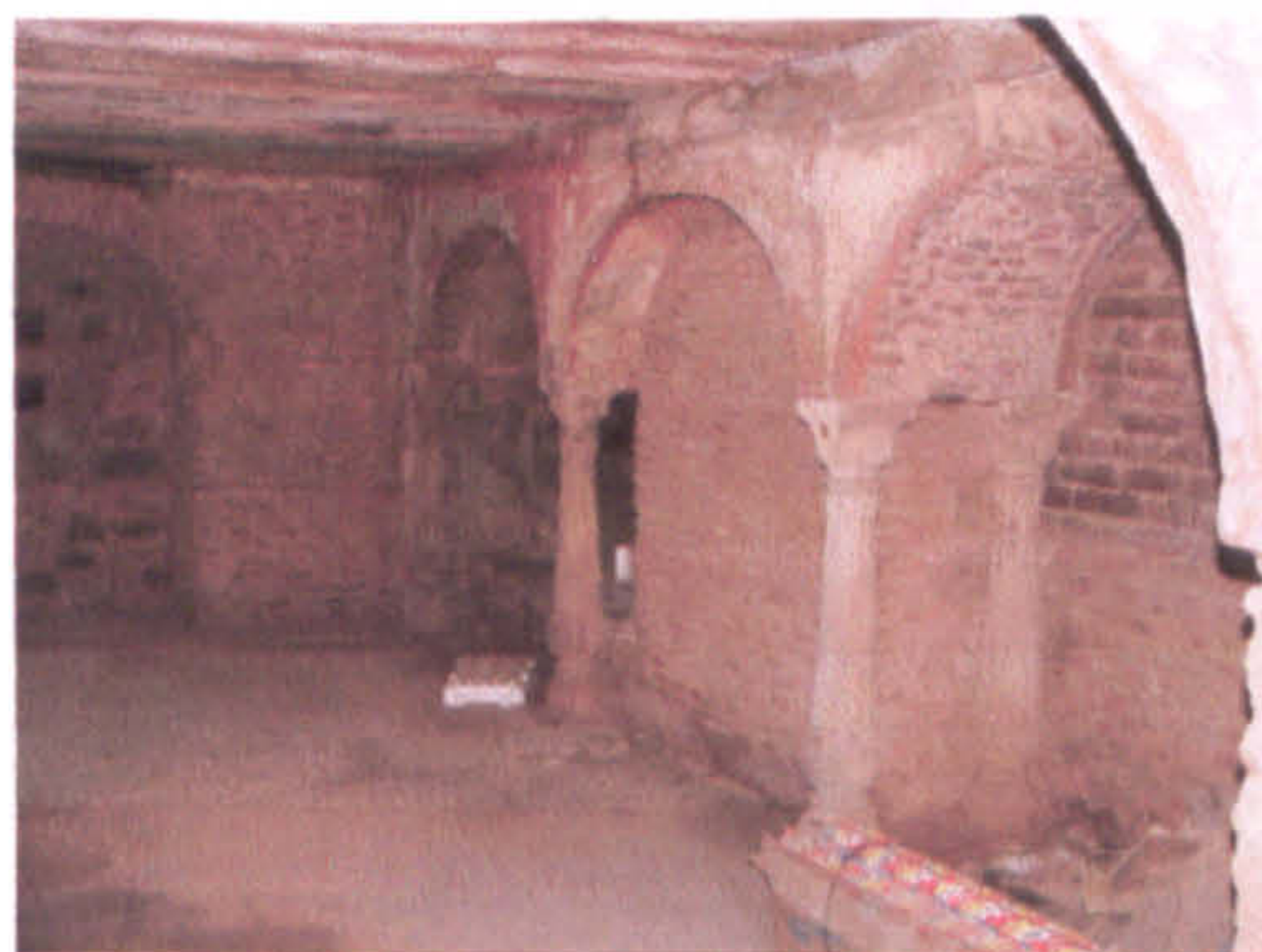
Fig.3.8h The Residency: interior of lower level chambers-I
