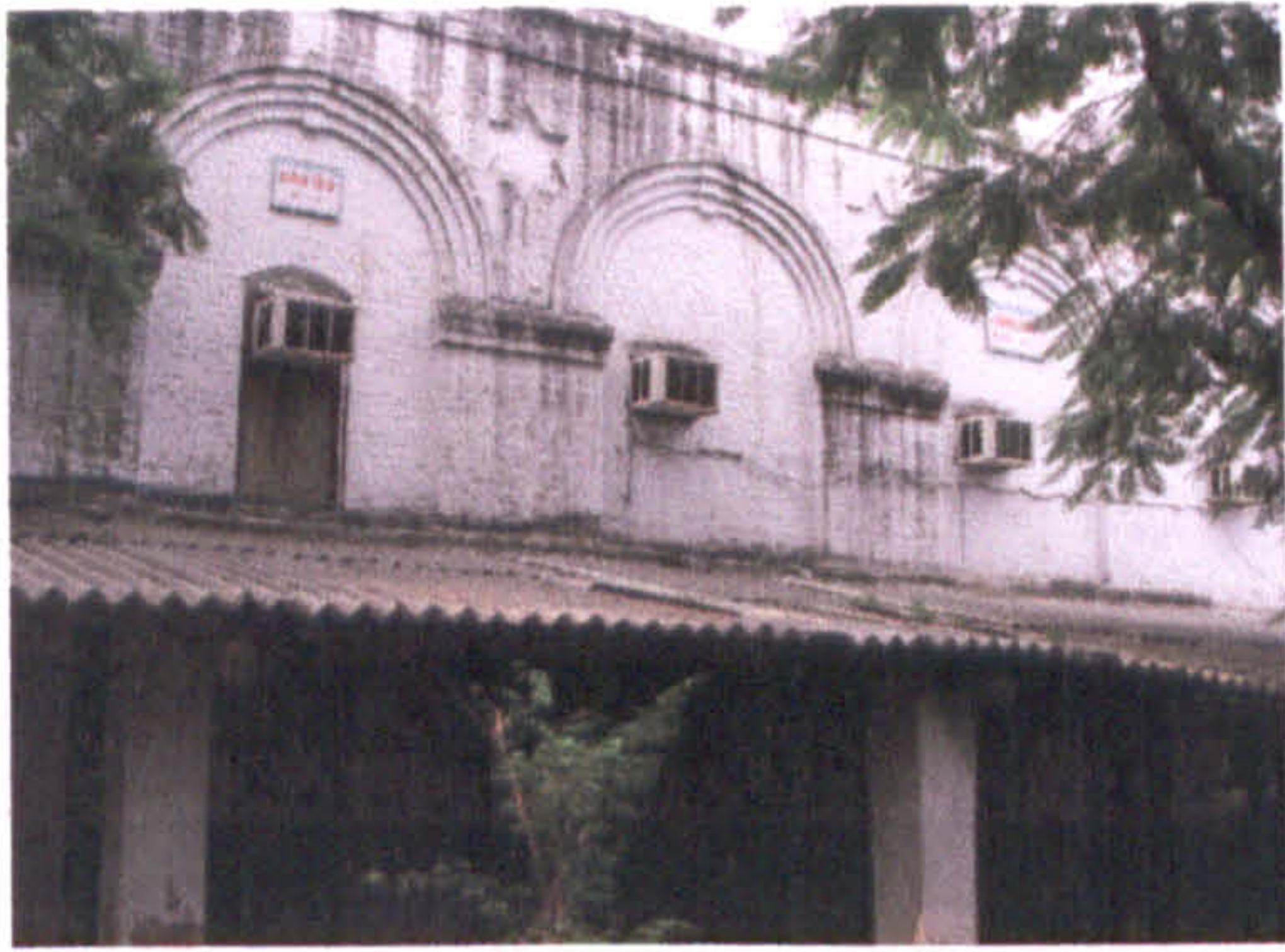
Fig. 7.14a The Baradari replaced by the Jamuna Hall
