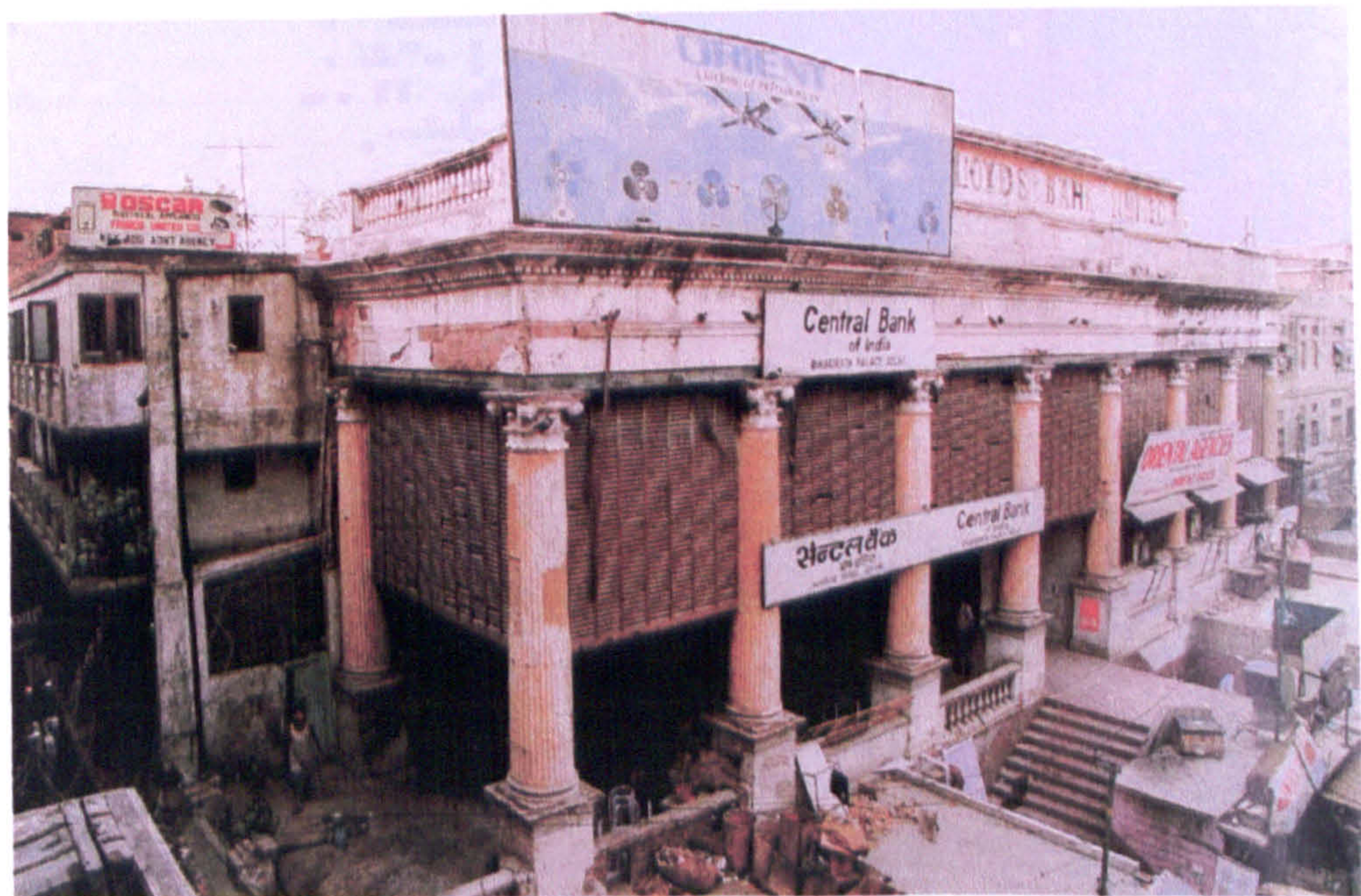
Fig.8.10b The Kothi as it stands today
