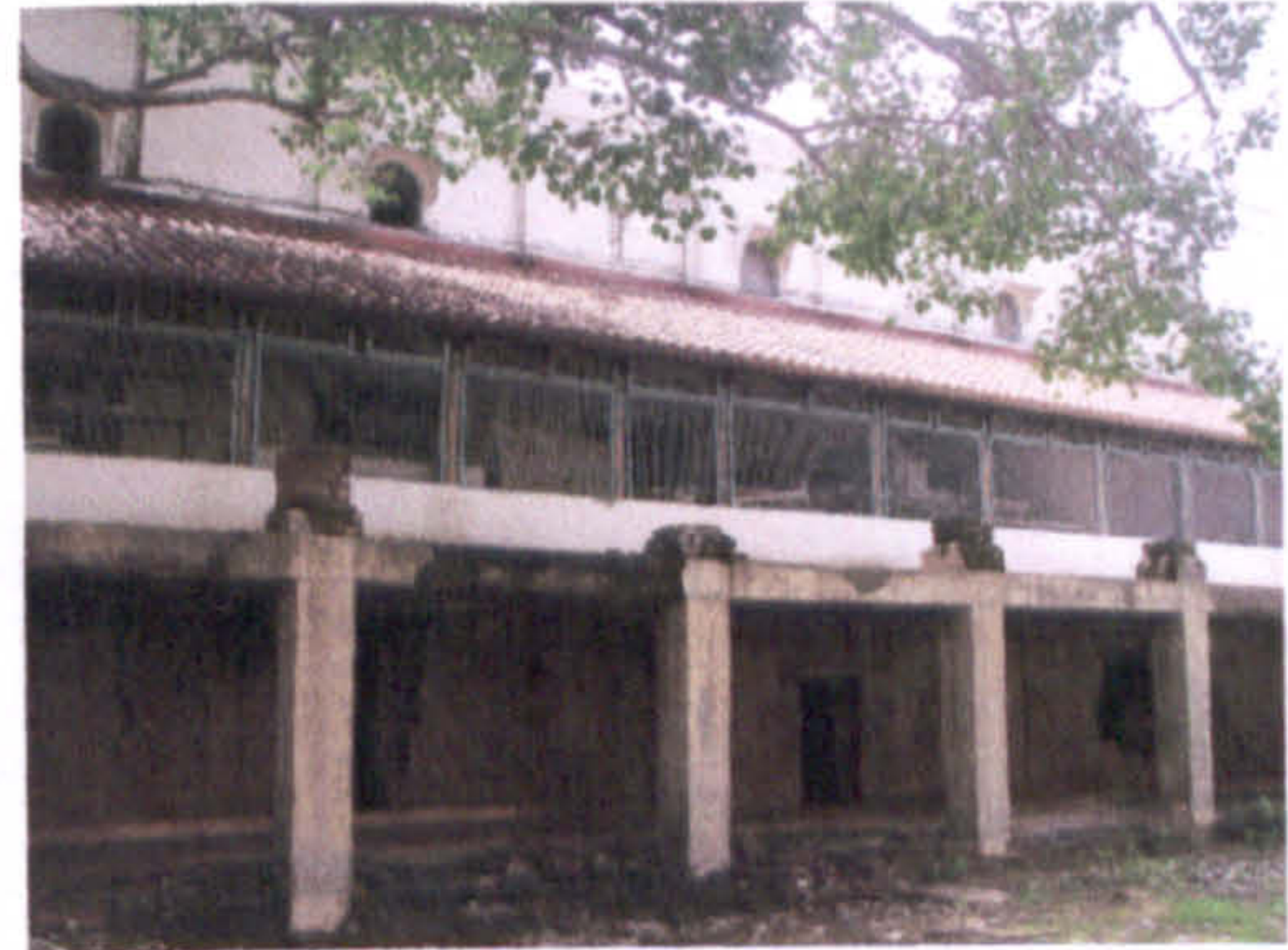
Fig.3.7b The Residency: rear verandah
