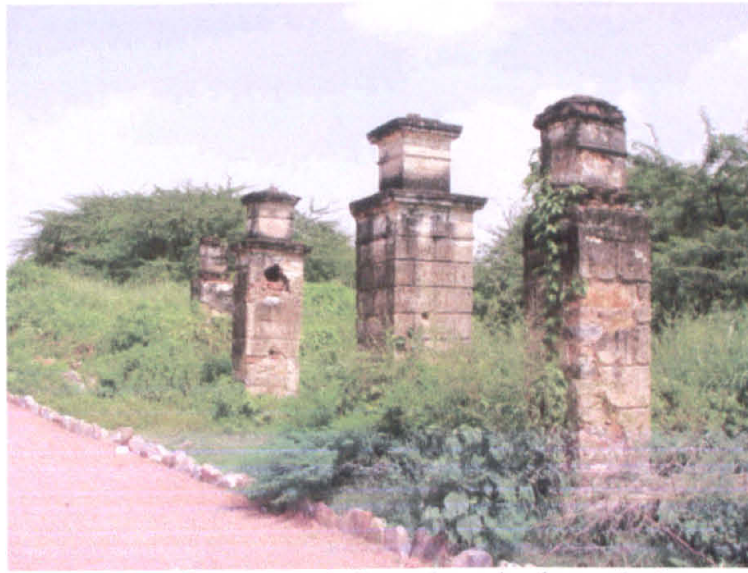
Fig.10.3c Gateposts delineating site boundaries
