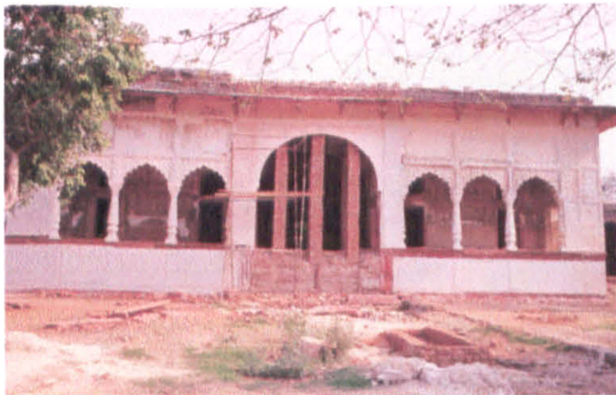
Fig.2.7b The Shish Mahal: front façade
