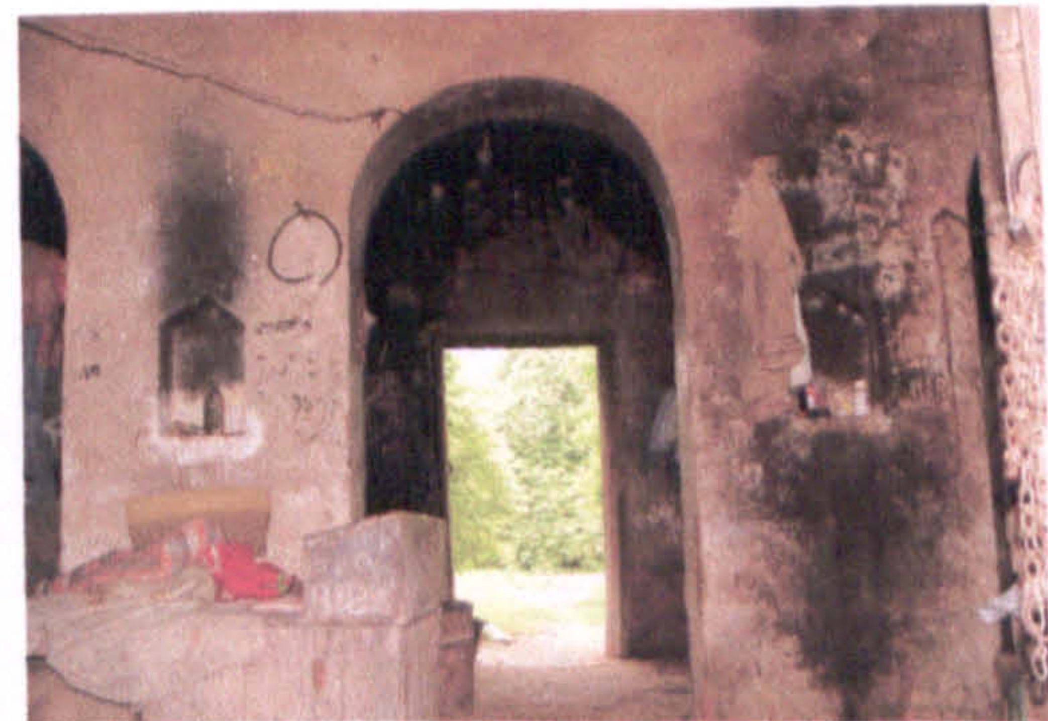
Fig.2.8b The service building: interior
