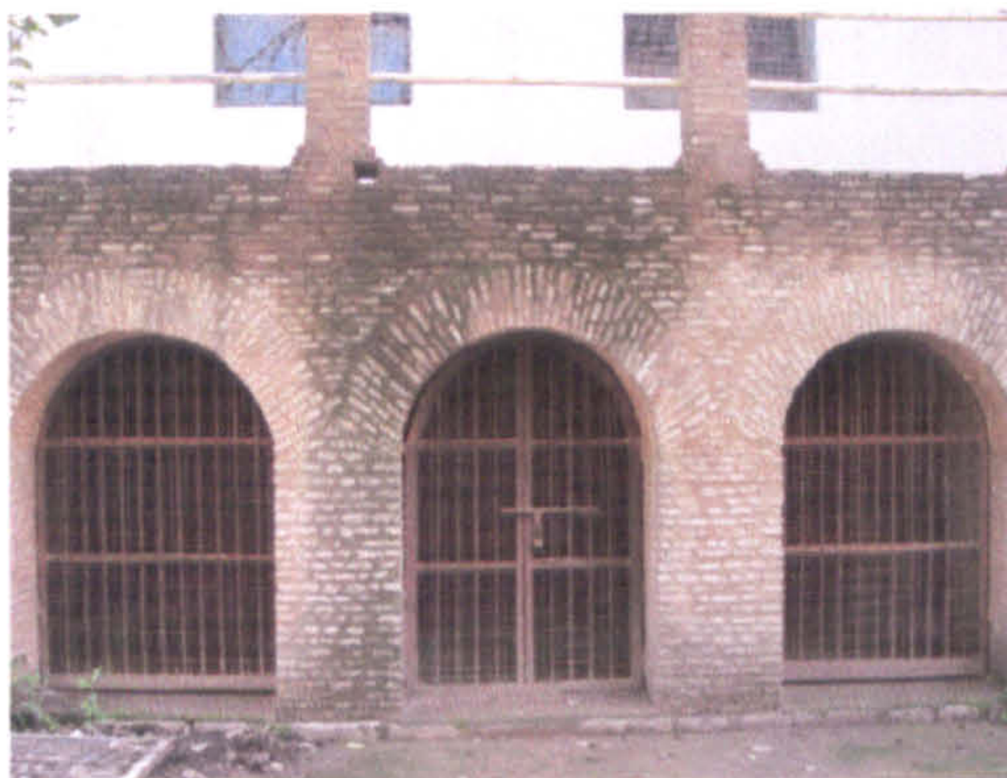
Fig.3.8f The Residency: lower level chambers-III
