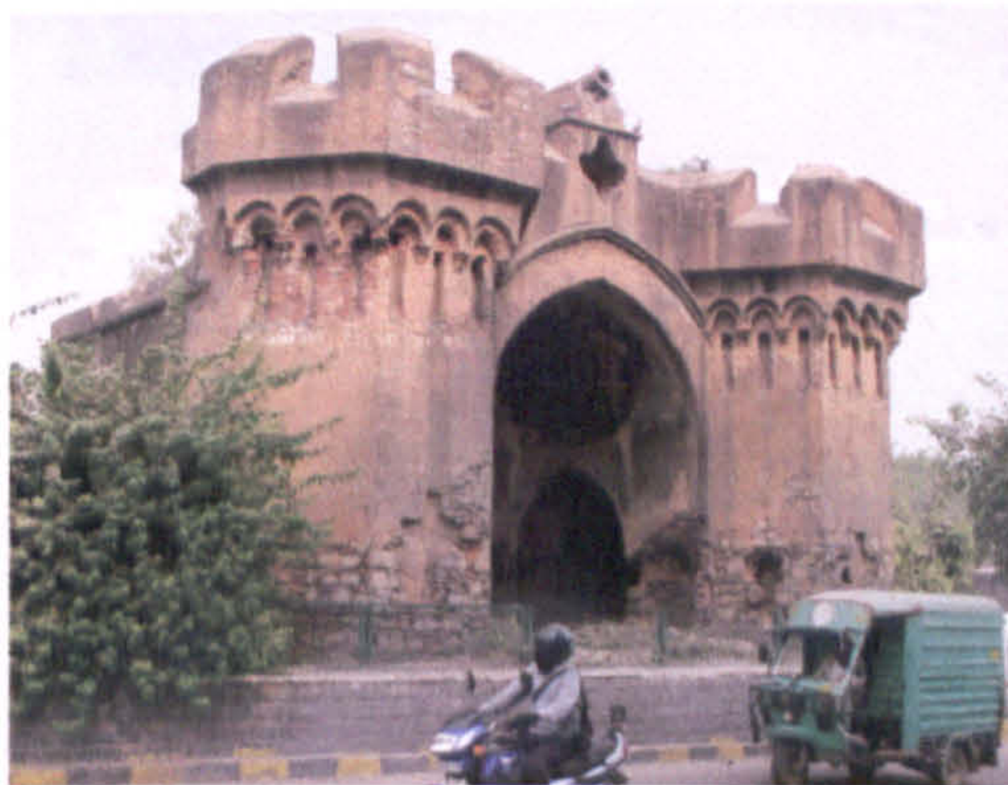
Fig.3.12 Remnants of the Magazine gateway damaged during the Siege
