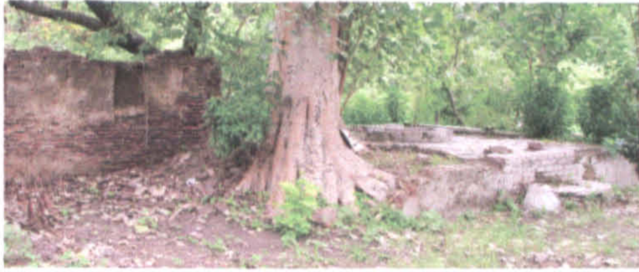
Fig.2.8c Ruins of an unidentifiable structure and a well
