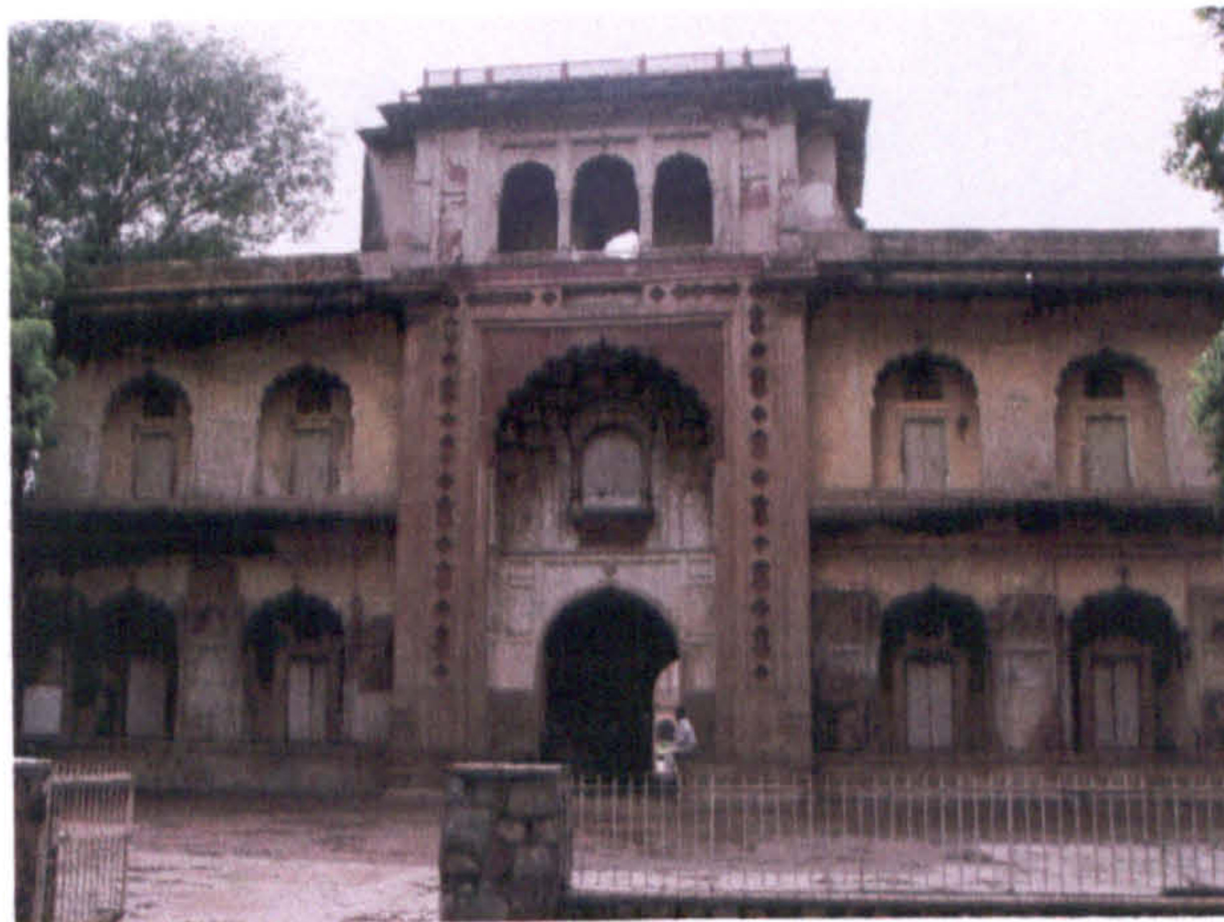
Fig.6.3 The entry portal on the east
