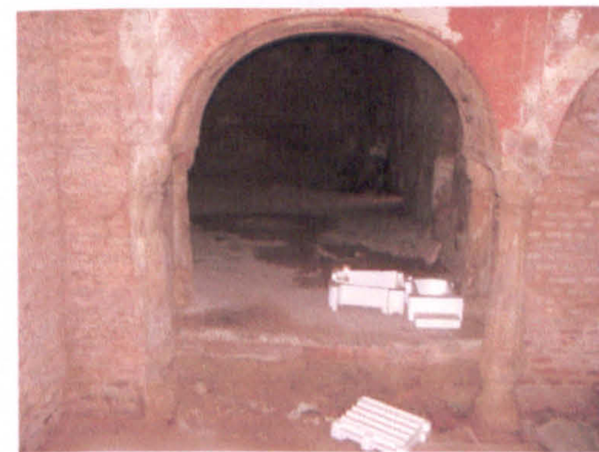
Fig.3.8i The Residency: interior of lower level chambers-II
