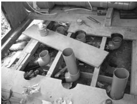
Figure 4.37: Three polyethylene pipes were buried at 0.5m, 1.0m and 1.5m.
