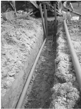
Figure 4.27: The PVC pipe buried at 1.0m depth is 50m long while the other pipes were only 30m long.
