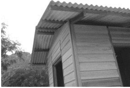
Figure 4.33: There is a gap under the roof for ventilation in the experiment shed. However, main purpose of building shed is for security of the equipment purposes.
