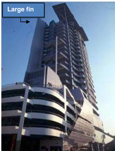
Figure 2.32: UMNO Tower in Pulau Pinang, showing the large fin or wing wind wall (Abdul Aziz and Mohd Adnan, 2008).
