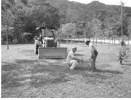
Figure 4.25: Construction work commenced.
