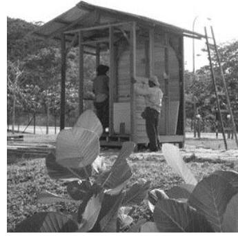
Figure 4.30: Progress in the experiment shed construction work.
