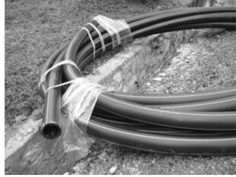
Figure 4.36: Polyethylene pipes were used to replace the broken PVC pipes.
