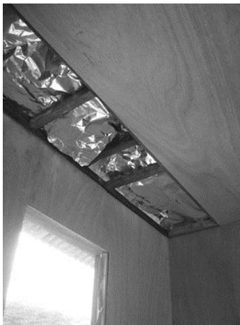
Figure 4.31: Ceiling construction in progress showing its insulation materials.
