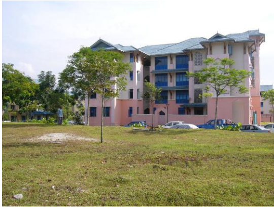
Figure 4.5: View of the site from South West before construction.
