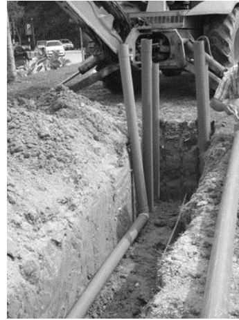
Figure 4.26: PVC pipes buried at 1.0m, 1.5m and 2.0m.
