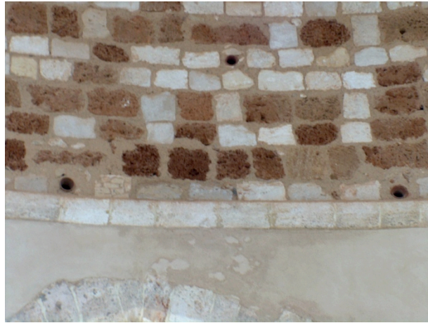
Figure 21 Photo of the clay embedded resonators
