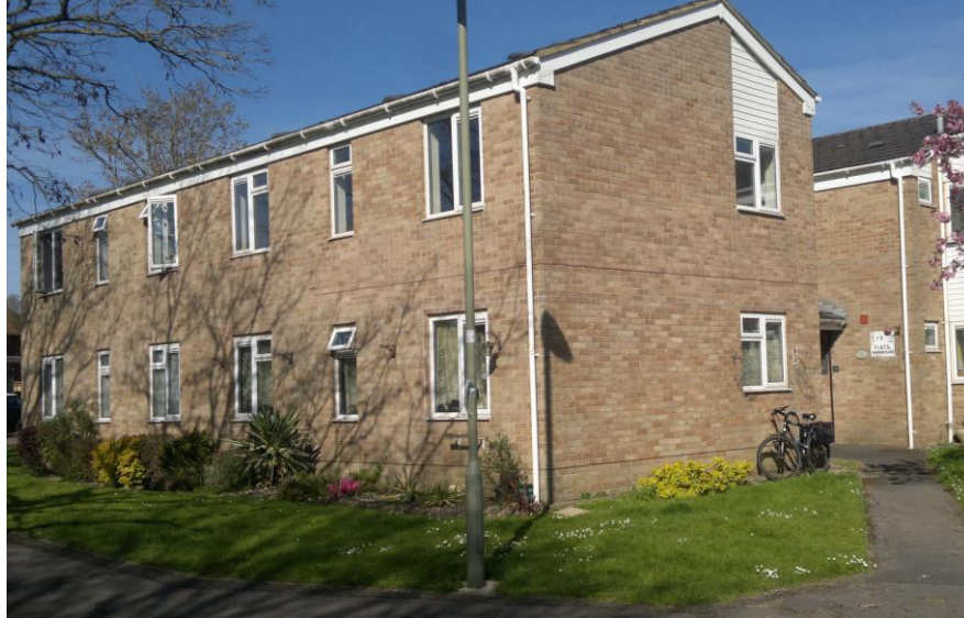
Fig. 8. Trial apartments with storage heating
