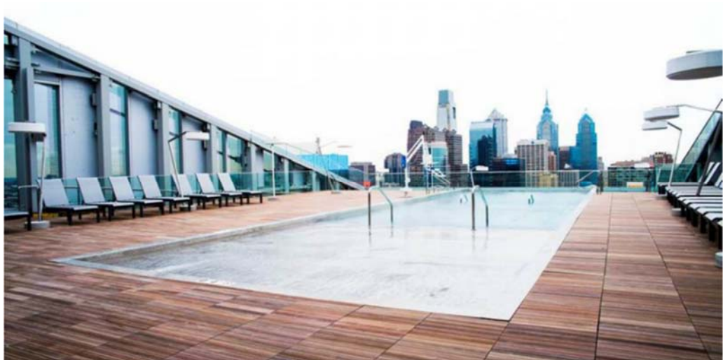
Fig. 9.15. Evo, Philadelphia, rooftop pool
