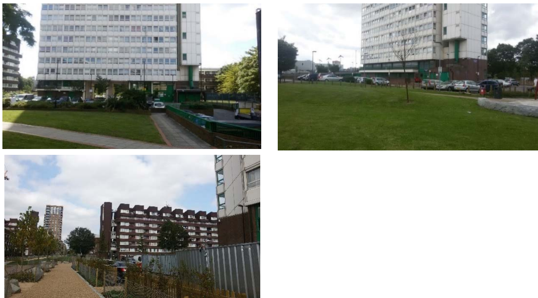
Fig. 5.5. Eddystone Tower: surroundings
