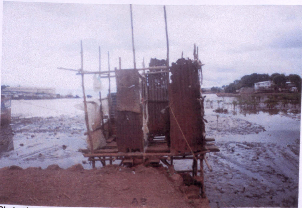
Photo shows hanging latrine (the only toilet facility available) in Kanikay, which empties directly in to the river or sea.
