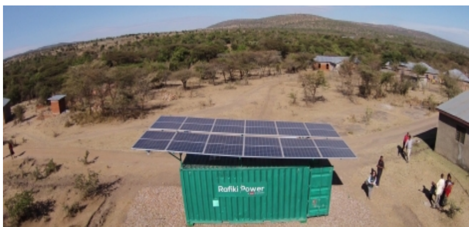
Figure 5.6: E.ON’s Rafiki Power PV-battery hybrid system in rural Tanzania (Source: eon.com)
