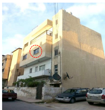
Photograph 2: The apartment, showing the window in photograph 1 circled. Source: Younis, 2015, unpublished
