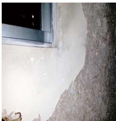
Photograph 1: The Japanese Plaster (teena yabaneyya) used by a low-income household. Source: Younis, 2015, unpublished
