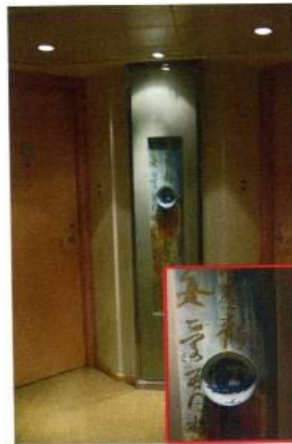
Figure 5.2 Jinling Hotel (photos taken in site survey)
