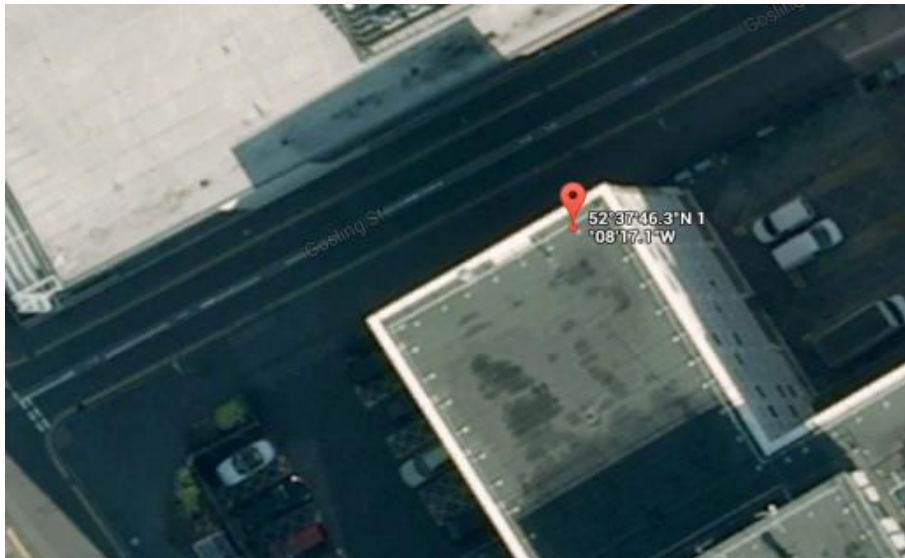
Figure 4.8 : Dry Riser Location: Lat: 52.629527, Long: -1.138096
