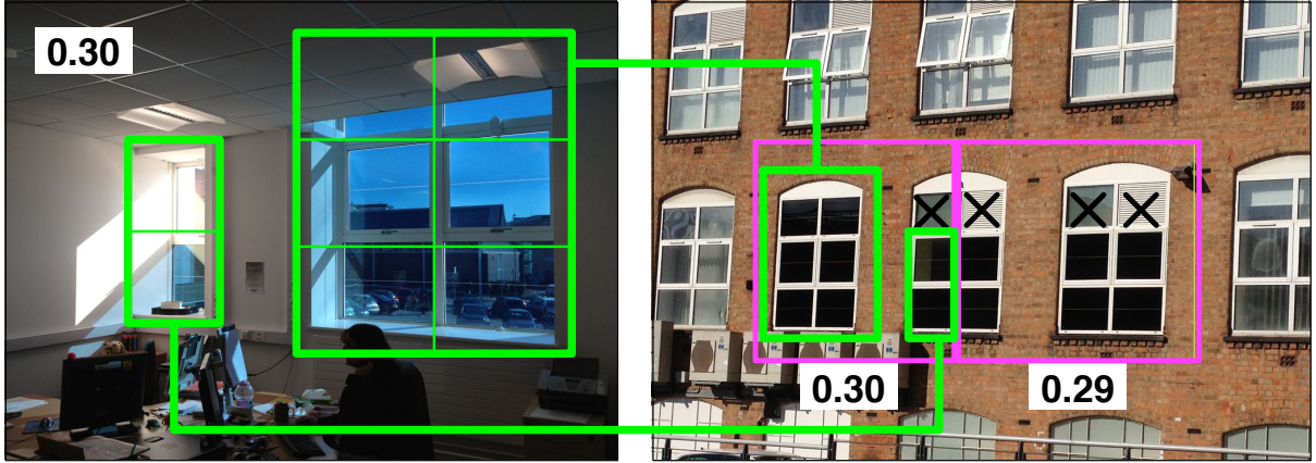
Figure 6: Photograph of Room 0.30 and the external facade.
