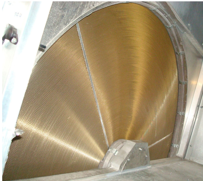
Figure 2.14: Epoxy coated HRW with anticorrosive material properties
