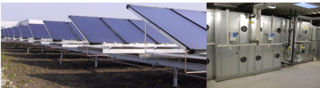
Figure 2.2: Solar collector array 1 (left) and investigated DEC-unit (right; Haller 2007)
