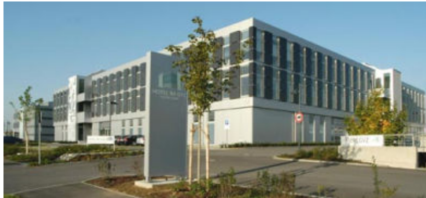
Figure 2.1: Multipurpose building in Ingolstadt (Haller 2007)
