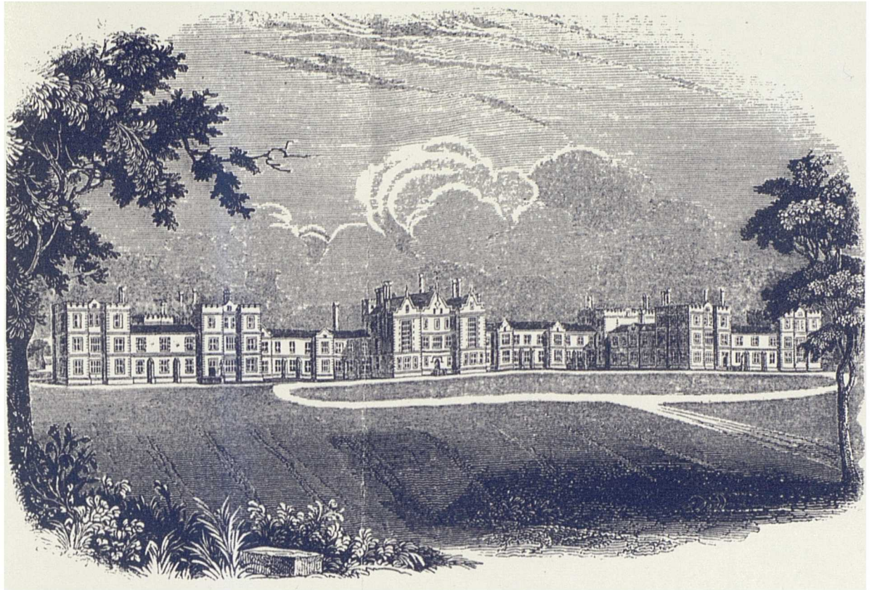
Plate 40. Wandsworth, London (1838-41). Engraving of entrance front and forecourt. A further example of the Tudor architectural style commonly used for asylum and workhouse buildings at this time, as well as for country houses (in The Mirror , 37 (13 February 1841), 1).
