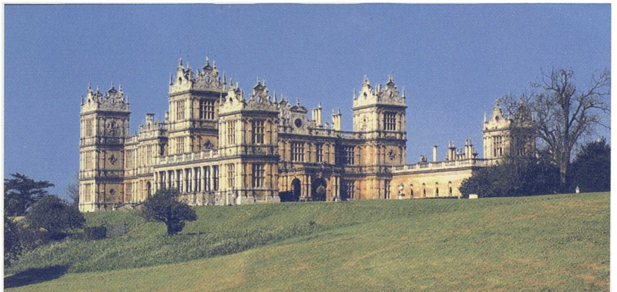
Plate 41. Mentmore, Bucks (1850s). House, in Jacobean style, and forecourt set on the terrace. The sunken service wing stands to the right of the dominant family wing. The windowless walls of the service wing (the position of windows is filled by niches) prevented servants overlooking arrivals, 2000 (SR).
