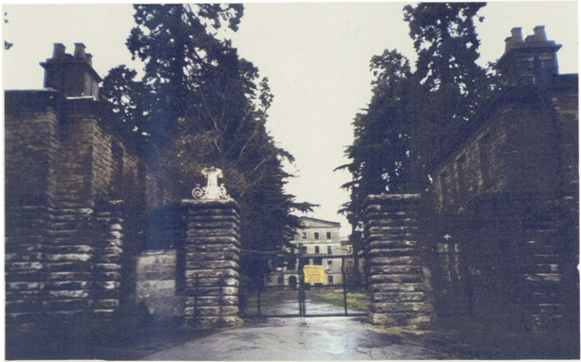
Plate 44. Maidstone, Kent (1830-33). Classical gateway at main entrance to estate, asylum building, and formal approach, 2000 (SR).
