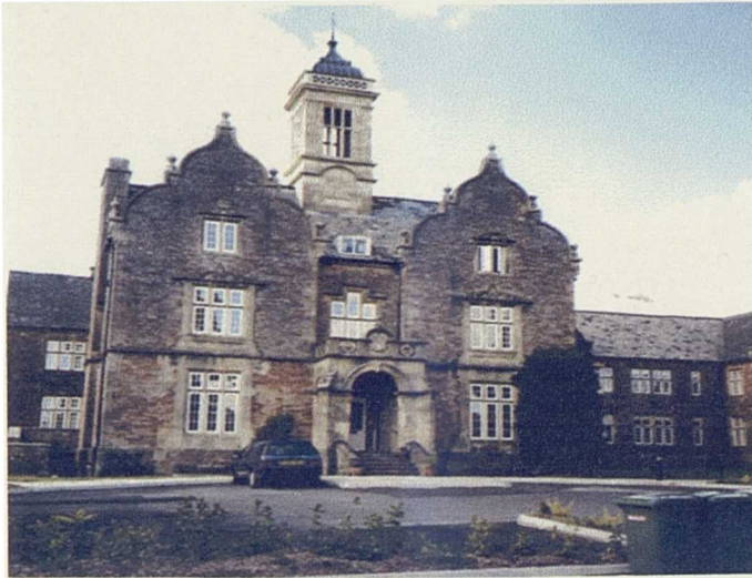
Plate 67. Wells, Somerset (1845-48). Visitors' entrance to the asylum building, in Jacobean style, 2000 (SR).
