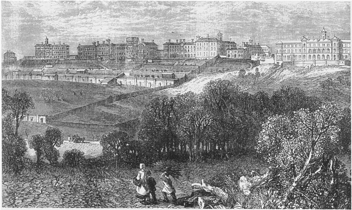
Plate 72. Broadmoor, Berks. (1860-63). Engraving of south front of asylum buildings. Terraces lead down from the male patients' blocks to the walled kitchen garden and asylum farmland in the foreground. Female block at far right, with smaller (two-storey) superintendent's residence separating male and female accommodation (in Illustrated London News (24 August 1867), 208).
