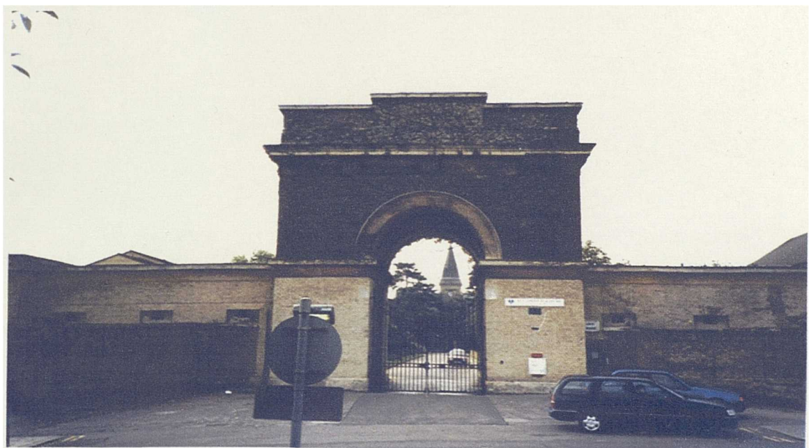
Plate 37. Hanwell, London (1828-31). Classical gateway and lodges at main entrance, 2000 (SR).
