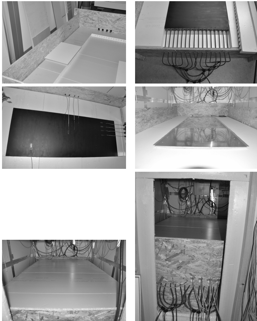
Figure F.2: More photos from the construction of the “ \epsilon -experiment”. top left: sizing the insulation layer surrounding the cold plate, top right: tubing on one end of the hydronic element, middle left: temperature sensors on the cold plate, middle right: hot plate installed on top, bottom left: last layer of insulation installed, bottom right: view from the outside of the chamber showing the experimental arrangement, tubing and sensor wiring.
