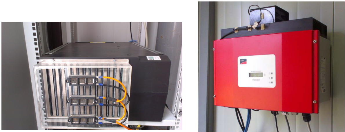
Figure 3-7: Heliocentris NEXA ™ 1200 fuel cell system (left) and SMA Hydroboy fuel cell inverter.
