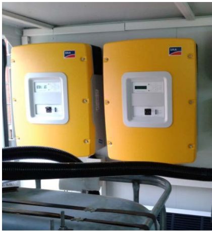
Figure 3-11: The left picture shows the two SMA Sunny Island 5048 inverter. To the right the picture shows the WAGO PLC and the LON Network Interface. Both installations are inside of the VRFB container.
