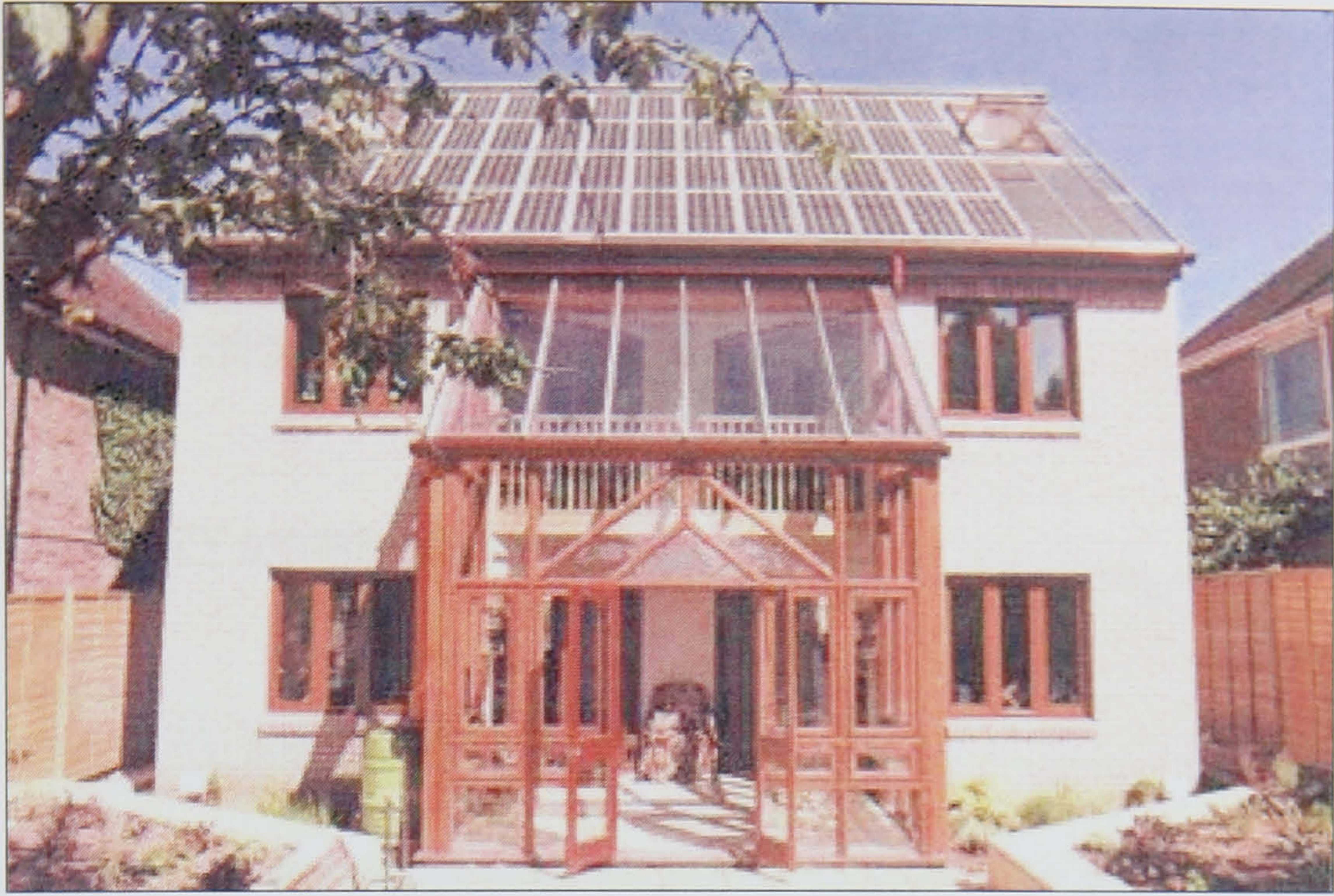
Figure 17. The Solar House in Oxford: grid-connected with PV system integrated into the roof. (From CIBSE, 2000.)
