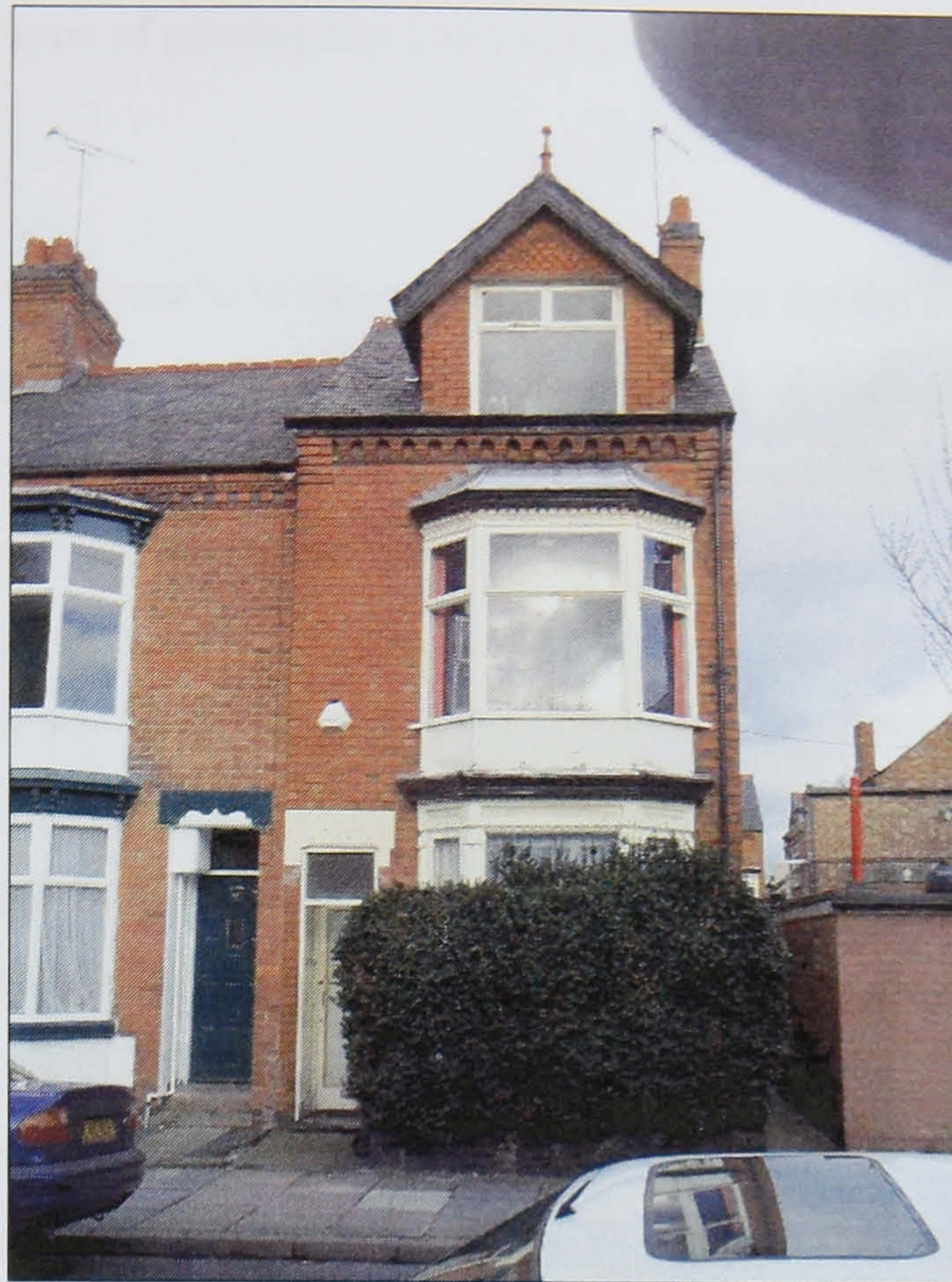
Figure 37. Room in the roof: implications for energy consumption and installation of active solar technologies.
