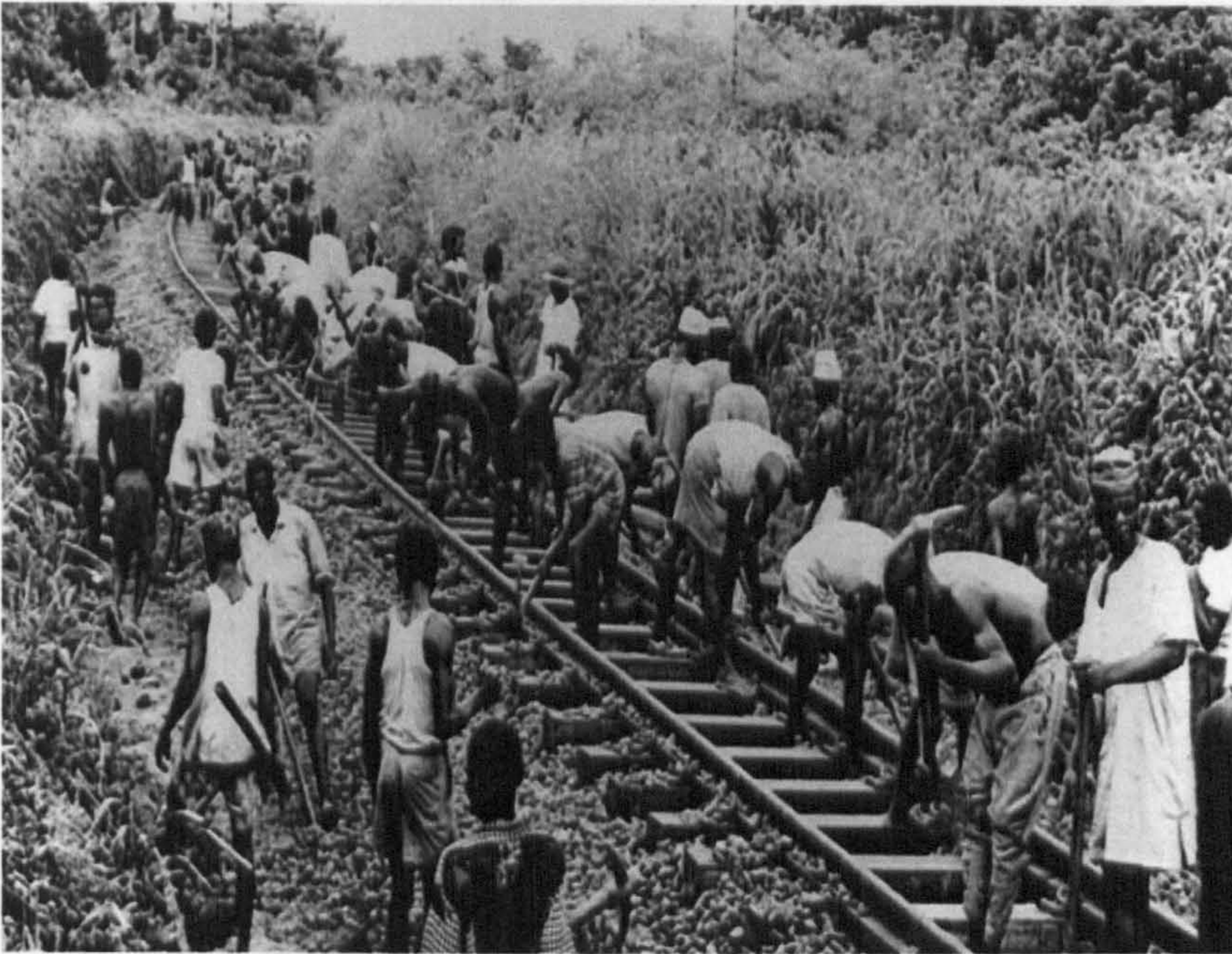
Figure 2.4.4.3: Labour intensive construction of the first Railroad in Nigeria
