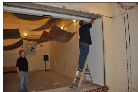
Figure 15.1 – The installation of a partition at Salford University
