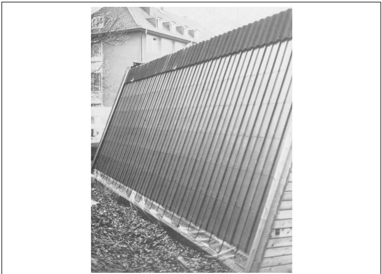
Figure 2.4: Typical Example of a Roof-Integrated, Unglazed Solar Absorber [14]
