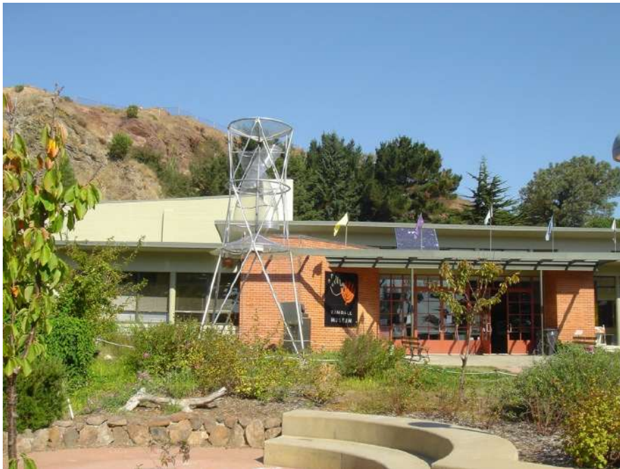
(d) Gound-mounted aeroturbine at the Randall Museum in San Francisco, California [Smith et al., 2012].
