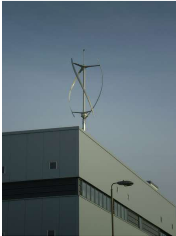
(a) A VAWT mounted on the roof of the Leicester City College, UK.
