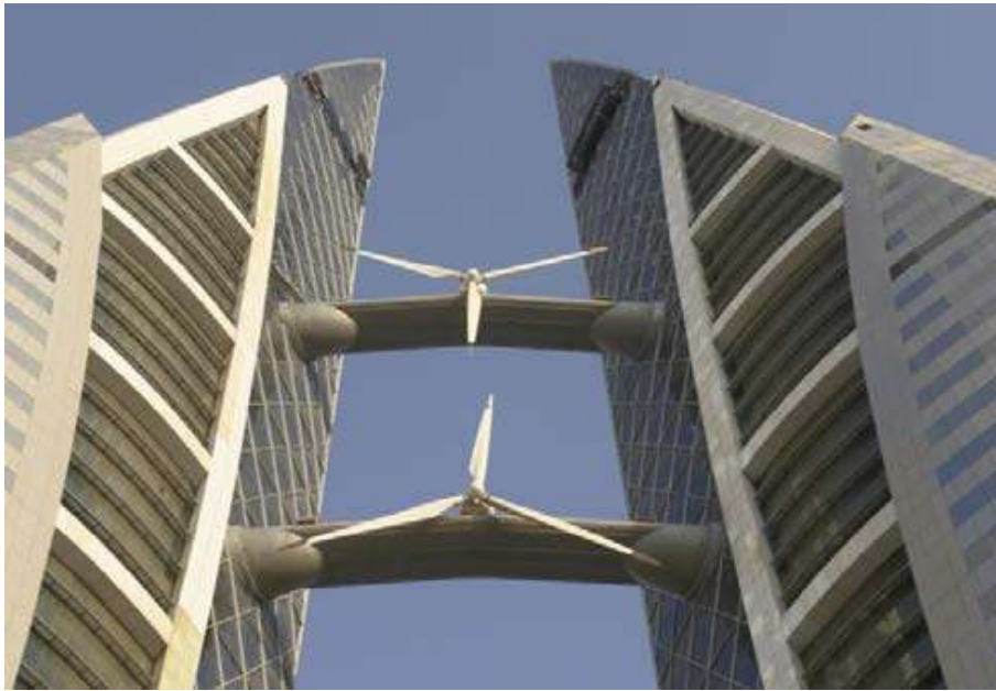
(c) Building-integrated wind turbine at the Bahrain World Trade Center [Smith et al., 2012].
