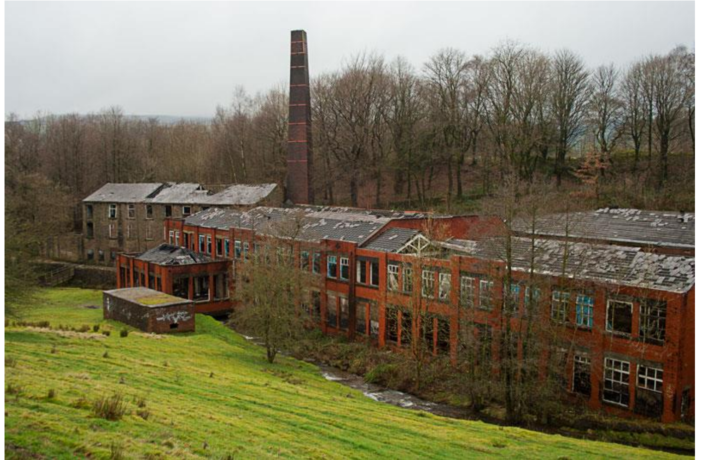
Rosebank Printworks (originally Edenwood Mill), Stubbins, Lancashire, 2012 ( www.derelictplaces.co.uk/ )
