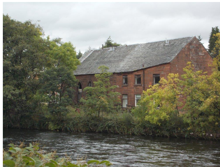
Dalmonach School House, at Dalmonach Works
