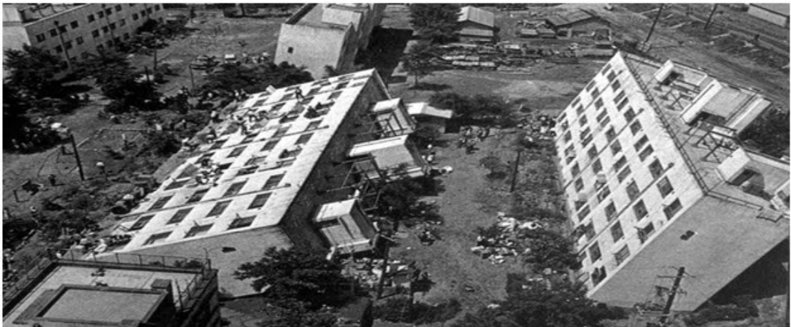
Figure 1 – Damage Resulting from Liquefaction Induced Ground Failure in the 1964 Niigata Earthquake
