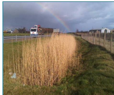
Figure 5 Trunk road wet swale which conveys and treats runoff, Scotland. Source: Alison Duffy
