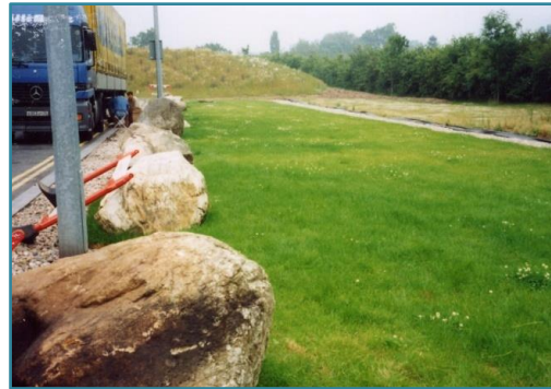
Figure 13 Vehicle lorry park, England. Sheet flow from the car park passes across the filter strip to the filter trench. Source: Fiona Napier
