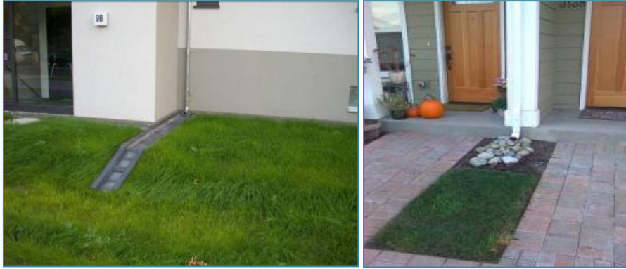
Figure 2 MDCIA exemplified for (a) housing in Berlin and (b) Seattle: roof runoff discharges onto front lawn. Foul connections are not an option.
