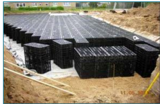
Figure 14 Geocellular units under construction. Source: Chris Digman
