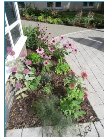
Figure 8 University courtyard, England - Porous paving / rain garden. Source: Alison Duffy
