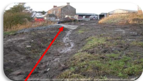
Concrete bund directs runoff away from a ditch to the left and into the newly constructed (unplanted) swale that transfers runoff from the yard
