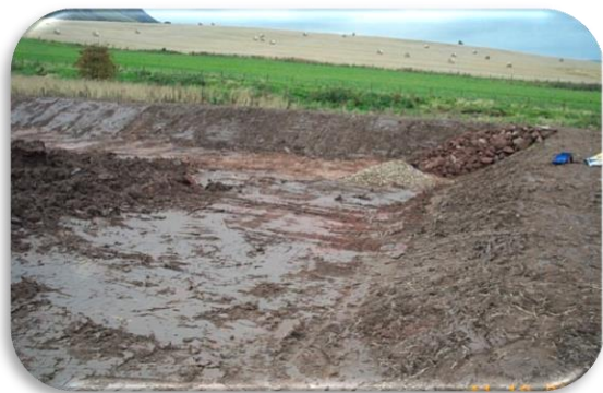
Excavation of the sediment trap bund 2004
