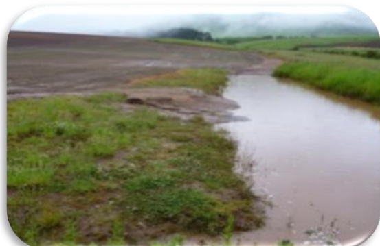
Sediment Trap Bund after heavy rainfall
