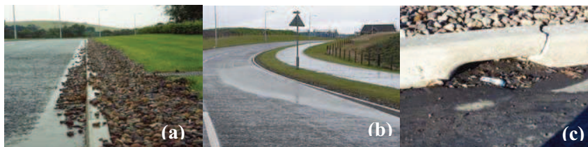
Figure 4: Problems with offlet kerb arrangements along Spine Road
