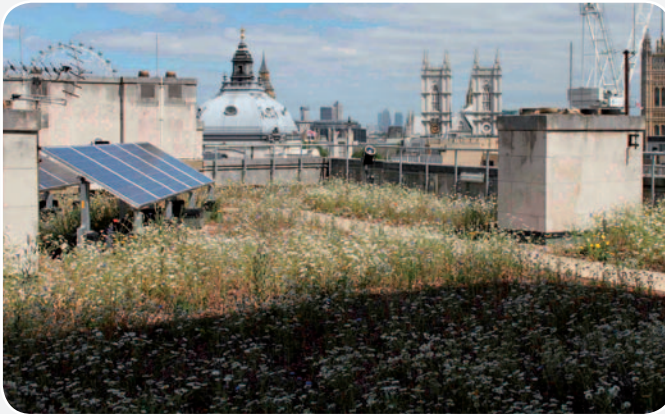
Figure 1 The biodiverse green roof of the Transport for London building on Broadway. Photo courtesy of Green Roof Consultancy Ltd.
