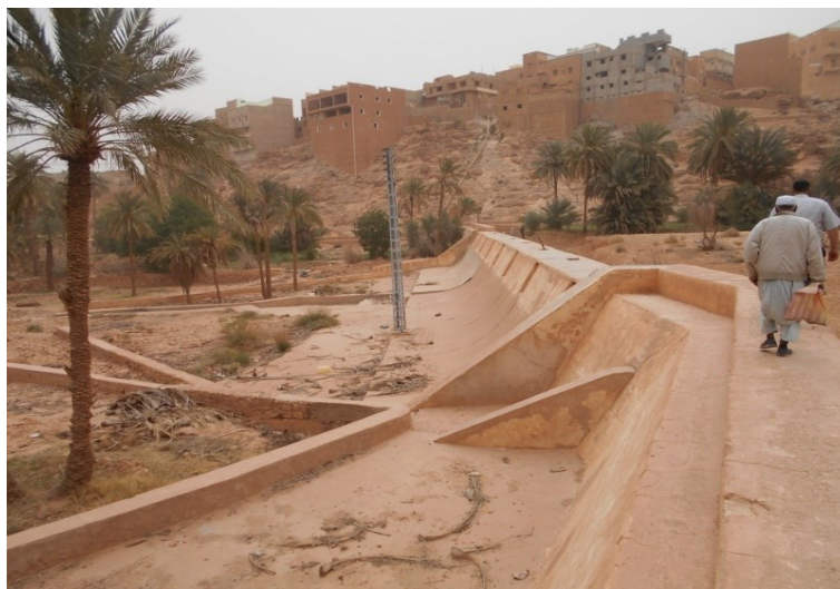
Figure 7. A view of the Ballouh Dam
