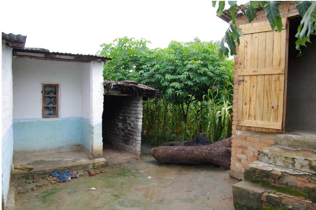
Photograph 2. Skyloo with tree removed and stairs
