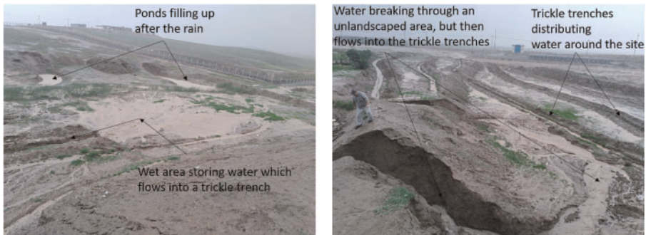
Figure 8 The SuDs-demonstration Site during the Floods of 22 and 23 November 2018
