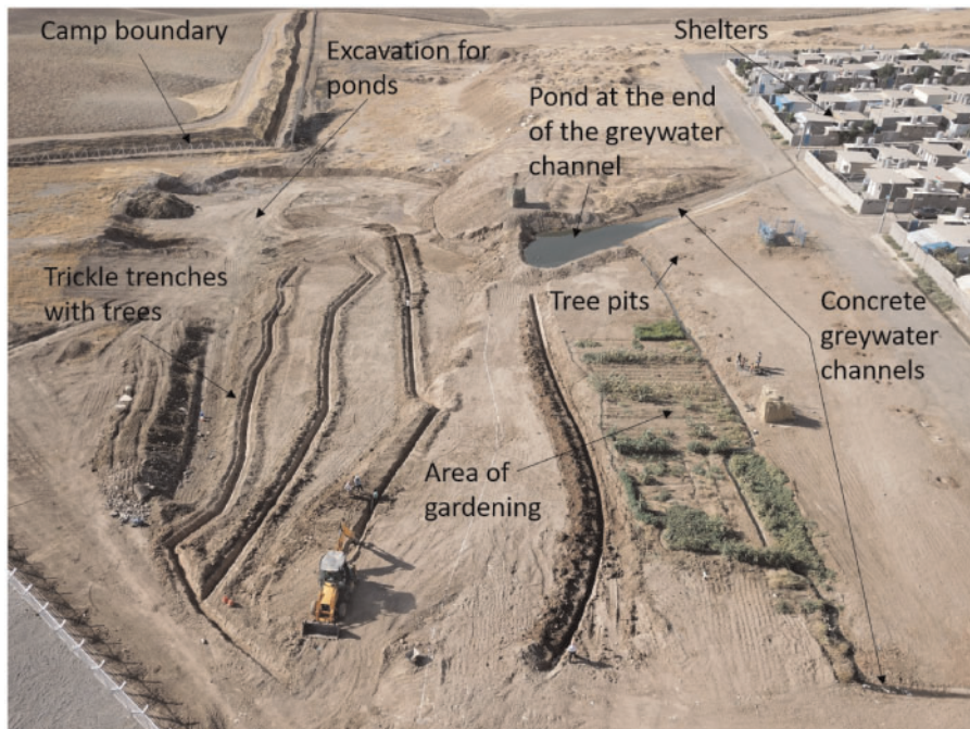
Figure 6 Aerial View of SuDS Site under Construction
