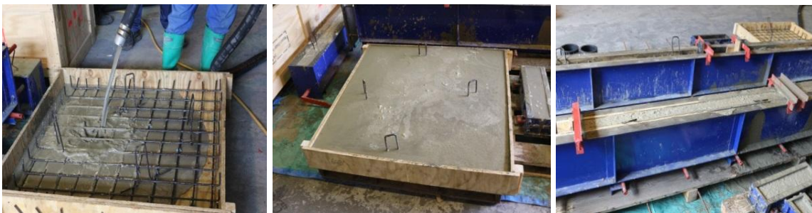
Figure 5: GEM-TECH material pumped into slab and beam moulds
