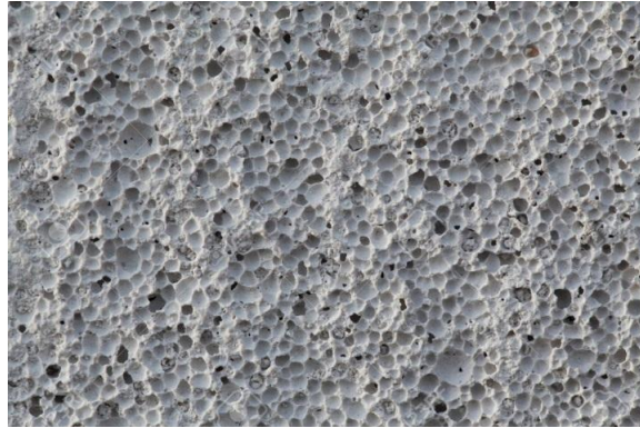
Figure 2: Aerated Concrete (Mohd Roji, 1997)
