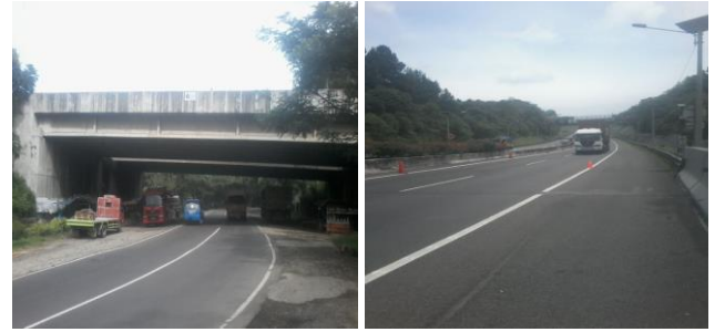
Fig. 4 The Cisomang underpass bridge
