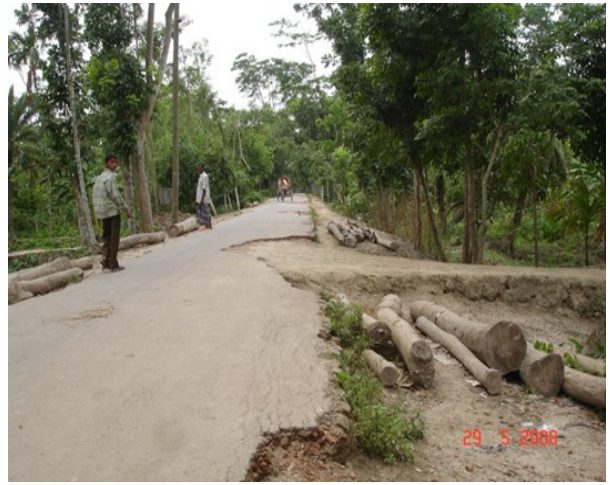
Figure 1: Storm surges breaks up the pavements of road network in Barguna district, Bangladesh
