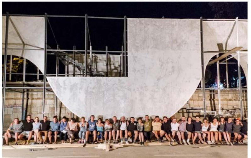
Figure 4. Construction process at the site
