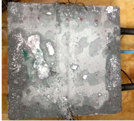
166 Fig. 1. Concrete specimen with Zinc Rich Paint (ZRP) primary anode
