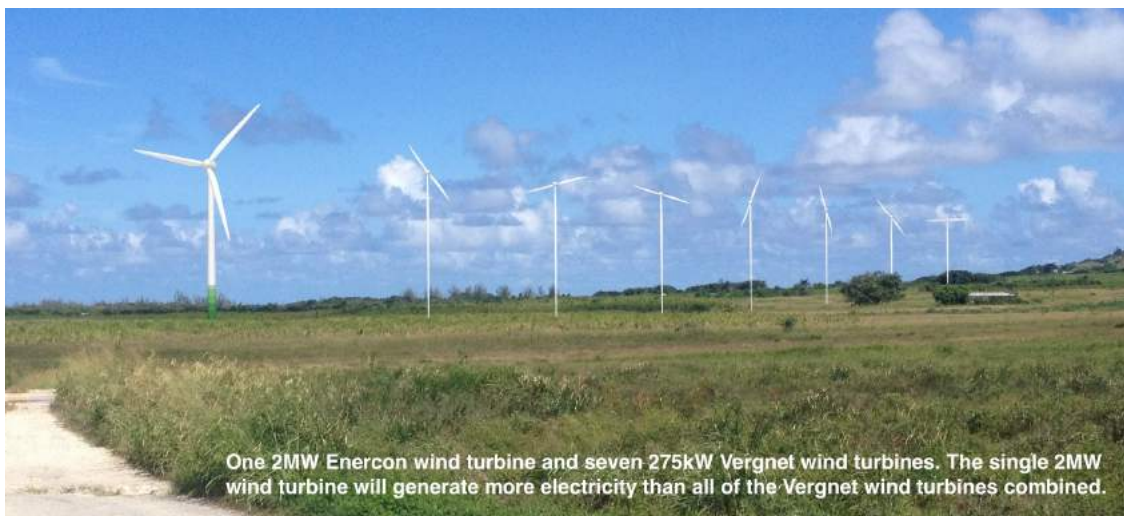
Figure 1. Photomontage of agricultural land in St Lucy, Barbados, highlighting the need for fewer larger wind turbines rather than many small wind turbines.
