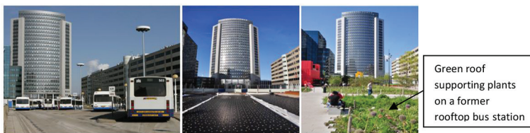
Figure 3. The roof park built on the former Orlyplein Bus Station deck , before, during and after construction.
