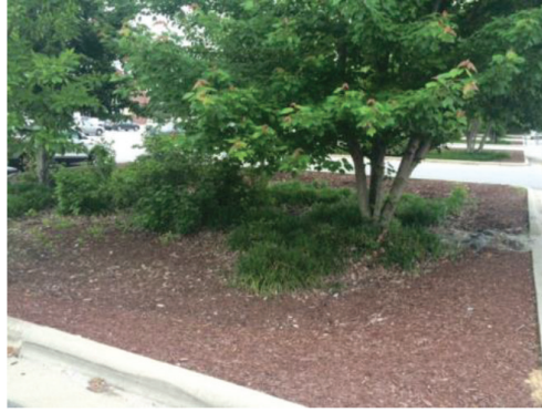
Figure 5. A bioretention cell with trees and shrubs in Raleigh, North Carolina, USA.
