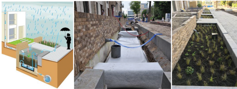
Figure 4. Left to right: Schematic of the green stream system, under construction and on the day of completion.
