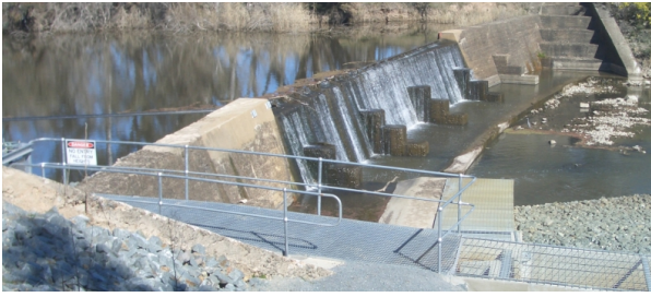
Fig. 2. Picture of Casey's Weir which is a free overfall weir with a fish ladder (seen in the foreground).
