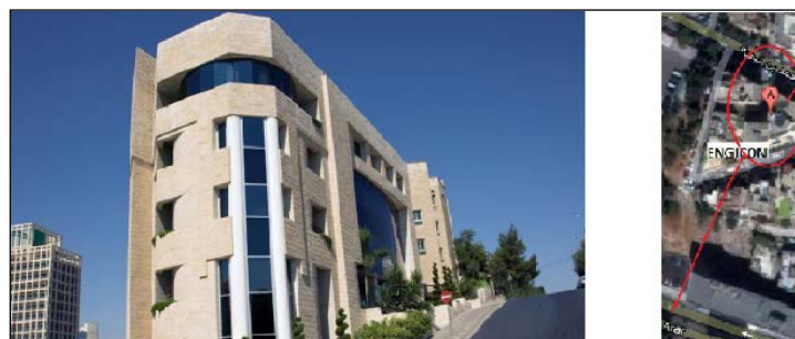
Figure 4: Certified building – Engicon office building and location map (Source: Engicon website)
