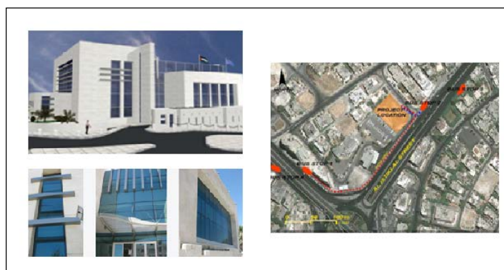
Figure 2: WHO building Gold Certified - External view and location (Source: Engicon report)
