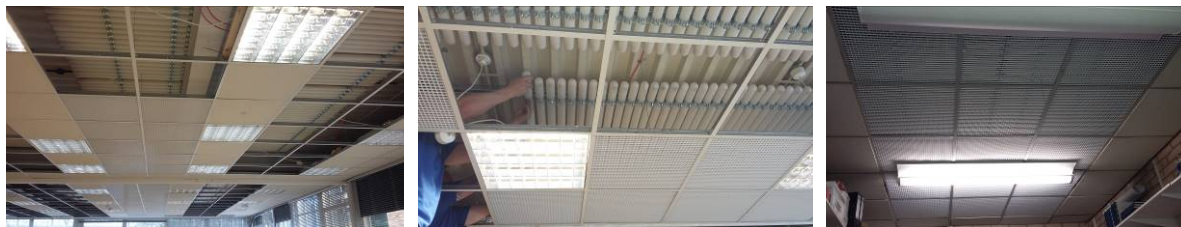
Figure 8: Installation of the PCM tubes
