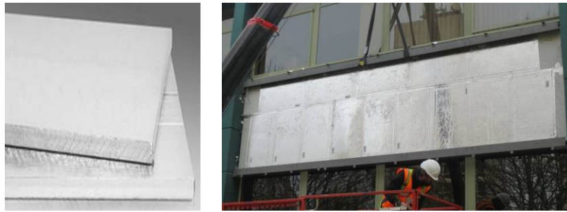
Figure 3. Image of a VIP and Final installation on-site
