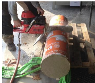
Fig. 5 : Cutting the puddingstone concrete column
