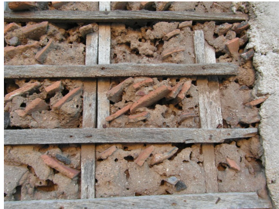
Figure 11: Close-up of infill material used in solid traditional bahareque in El Salvador – note the pieces of clay tiles added to the soil (Kaminski, 2016)
