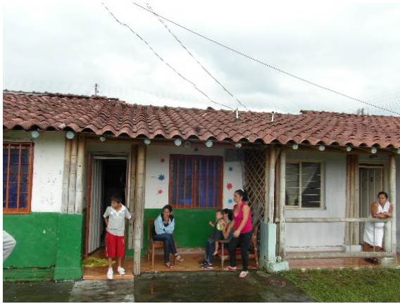
Figure 18: Post-earthquake engineered bahareque housing in Barcelona, near Armenia (Kaminski, 2016)
