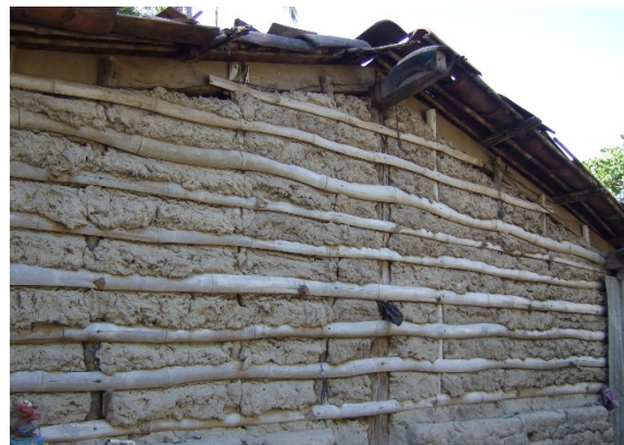
Figure 4: Traditional rural bahareque housing in El Salvador. No outer render has been applied (Kaminski, 2016)
