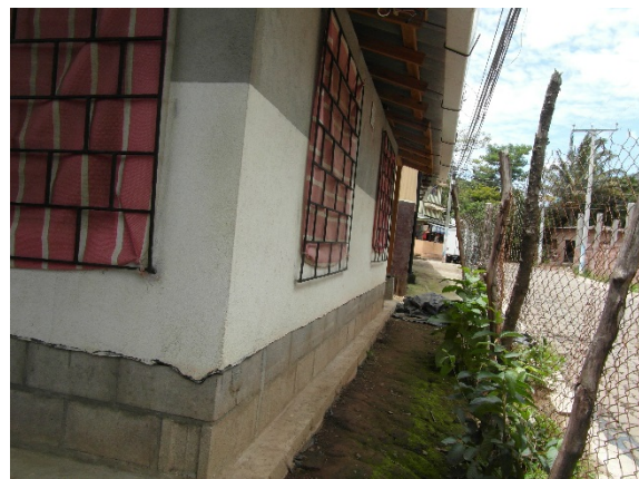
Figure 27: Cane and timber housing, El Salvador – complete. Note the upstand, damp-proof membrane and large overhang, all protecting the wall from moisture and rain (Kaminski, 2016)
