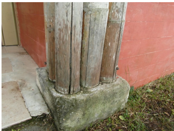
Figure 38: Fungal damage, splitting and bleaching of boron-treated bamboo exposed to the sun and rain after around 10 years, Colombia (Kaminski, 2016)
