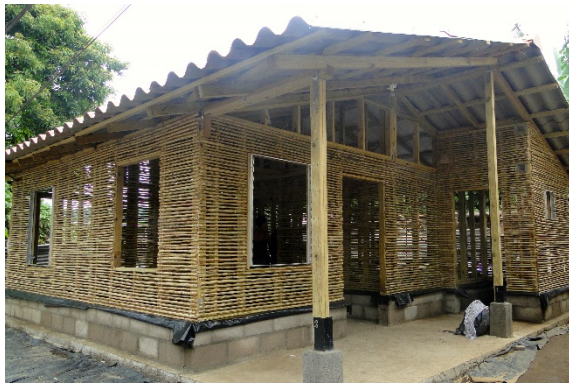
Figure 24: Cane and timber housing, El Salvador – before application of render. Note the large overhangs on all sides and the elevated frame on a damp-proof membrane (Kaminski, 2016)
