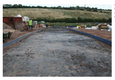
Figure 120 Sprayed surface of stabilised soil before constructing the paste layer
