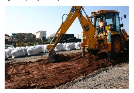
Figure 108 Levelling the spread soil using the JCB
