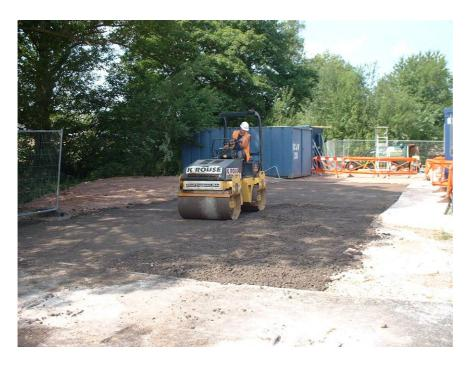
The completed layer of RRC is shown in Figure 102. The surface of the concrete was sprayed with a bituminous emulsion layer to prevent evaporation of water up to 28 days curing.
