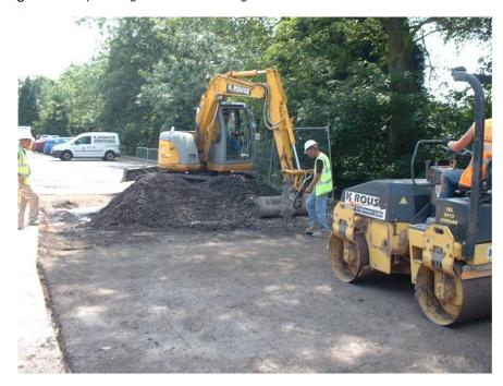
Figure 101 Concrete compaction using a 3-tonne vibrating roller
