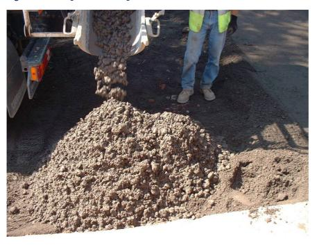
Figure 99 Placing and spreading the last batch of concrete
