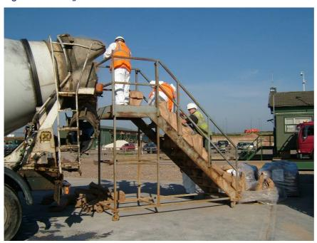
Figure 97 Loading blended binder bags into the truck mixer
