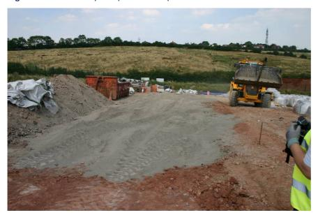
The mixture of soil and powder was blended using a rotavating blending machine as shown in Figures 112–114. The powerful and heavy blade of the machine provided a homogeneous blend of soil and binder along the road.
