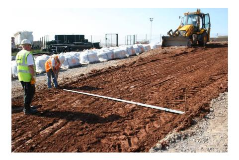
The blended powder was then spread over the area using a volumetric method. To achieve the required amount of binder per cubic metre of the compacted soil, 150 mm of the blended powder was spread over the trial area manually and using the JCB. Figures 110 and 111 show the placing and levelling of the powder on top of the level soil.
