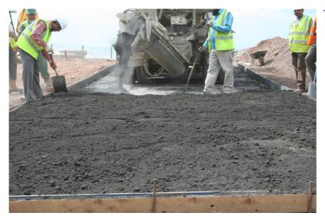
Figure 122 Spreading and levelling the semi-dry paste
