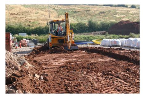
Figure 109 Controlling the accuracy of the thickness of spread soil
