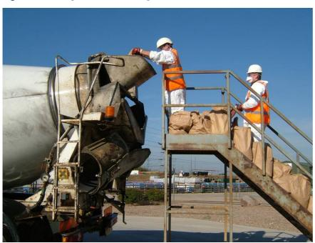
The mixture of aggregates, water and blended binder was mixed thoroughly in the truck mixer for about 10 minutes before being delivered to the site.
