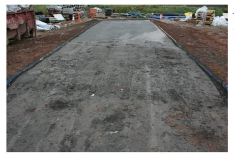
Figure 124 Finished surface of the compacted semi-dry paste
