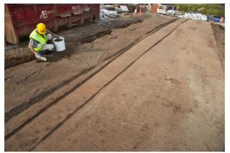
Figure 118 Finished surface of the stabilised soil
