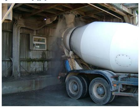
After mixing the aggregates and water thoroughly for about five minutes, the blended binder was loaded manually into the truck mixer. It had been planned to load the blended binder into the truck mixer using an auger system but a scheduling problem meant that the binder had to be loaded by hand (Figures 96 and 97).
