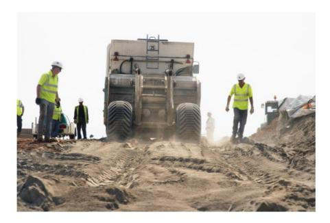
Figure 113 Rotavator in blending position
