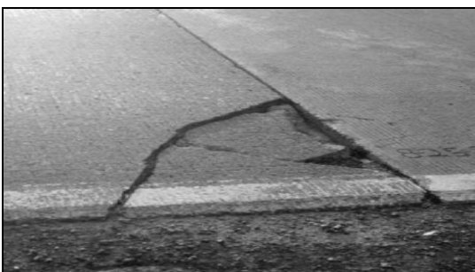
Figure 11. Warping failure
